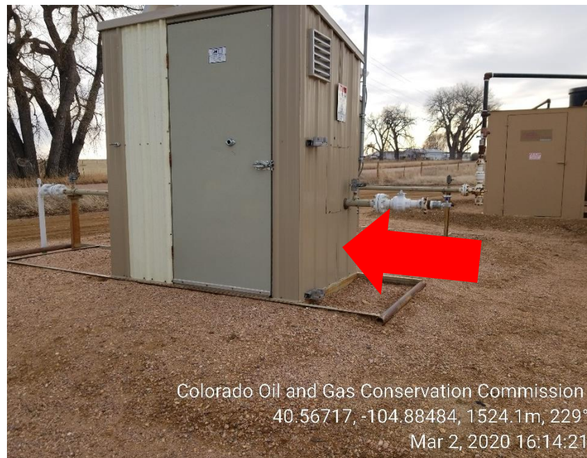
Photo 16: Unused/disconnected gas meter
