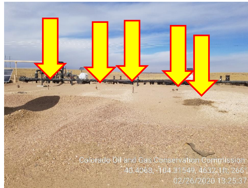
Photo 6 – Unmarked Risers and Stained Soil West of Compressor
