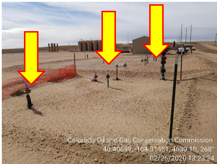
Photo 5 – Unmarked Risers East of Gas Lift Meter House
