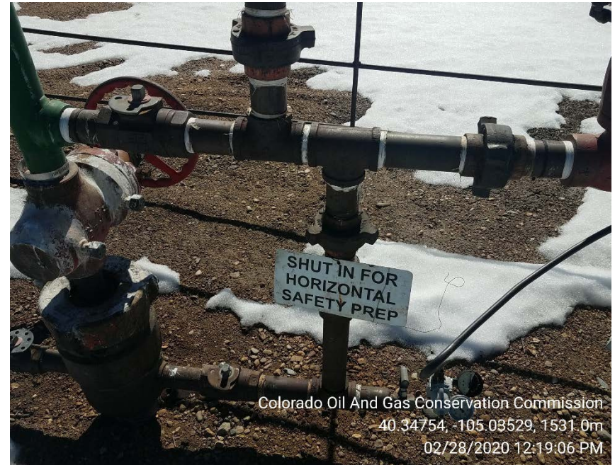
HZ safety prep sign
