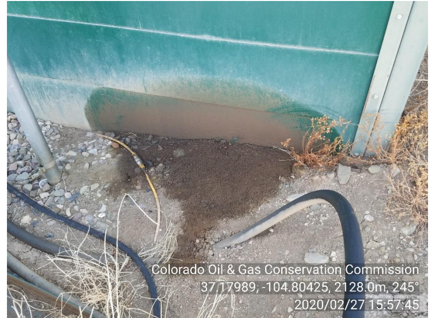
PHOTO 12: IMPACTED SOIL NEAR SOUND WALLS BETWEEN COMPRESSOR SKID AND SOUND WALL. Conduct maintenance on equipment, cleanup stained material and review self inspection processes. CA DATE 3-3-20.
