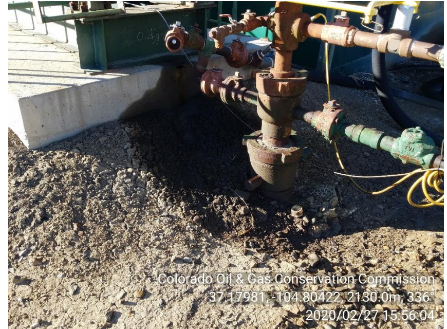
PHOTO 10: IMPACTED SOIL STARTING FROM PUMPJACK PAD AROUND WELLHEAD. Conduct maintenance on equipment, cleanup stained material and review self inspection processes. CA DATE 3-3-20.
