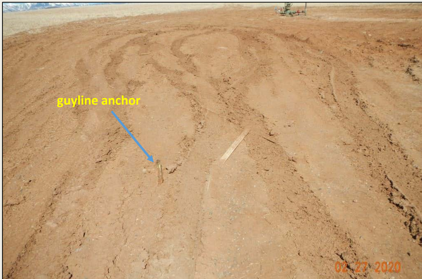
Photo 6. View of guyline anchor at well pad entrance where marker is no longer functioning, needs to be marked or removed.
