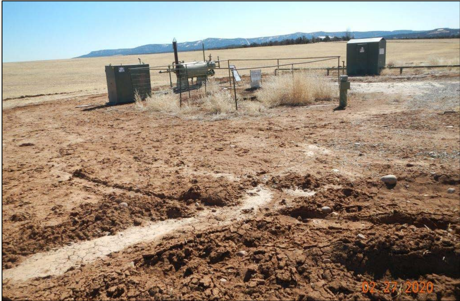
Photo 5. View of facilities in the southeastern project area. Lighter colored soil in flow pattern toward facilities and beyond, appears to be from release.
