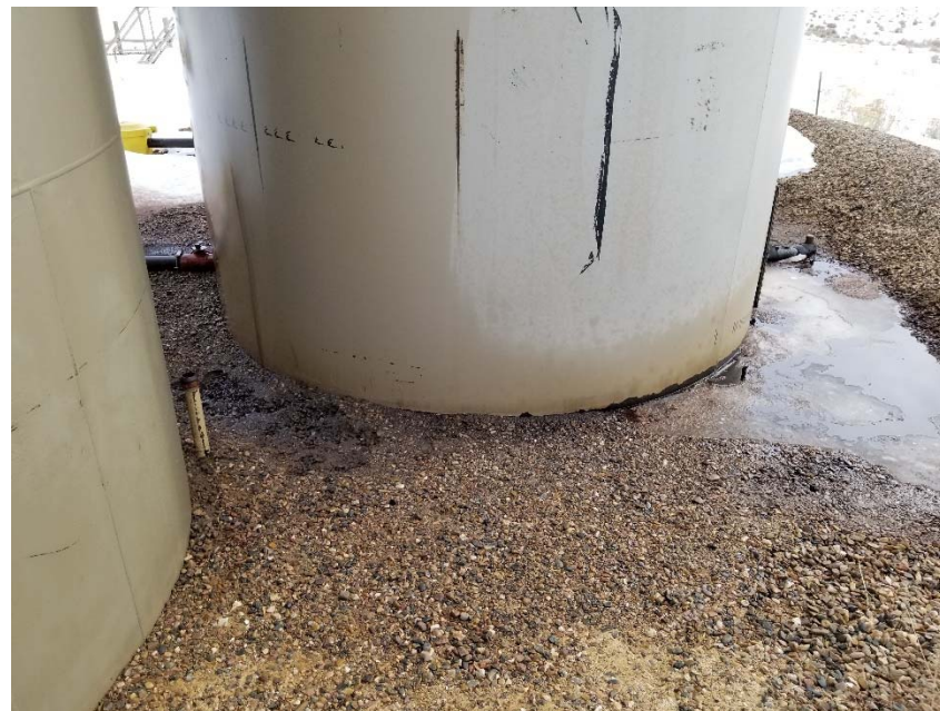
Photo 8. Stained soil and free product around base of tanks.
