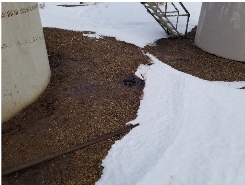
Photo 7. Stained soil and free product around base of tanks.
