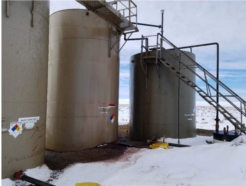
Photo 1. Stained soil and free product around base of tanks.
