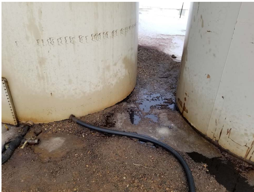
Photo 5. Stained soil and free product around base of tanks.
