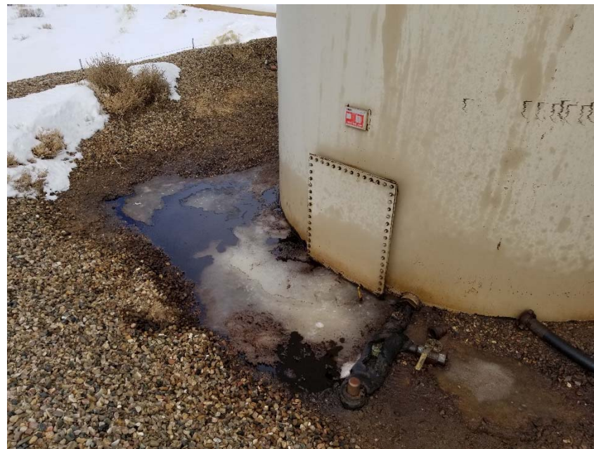
Photo 6. Stained soil and free product around base of tanks.
