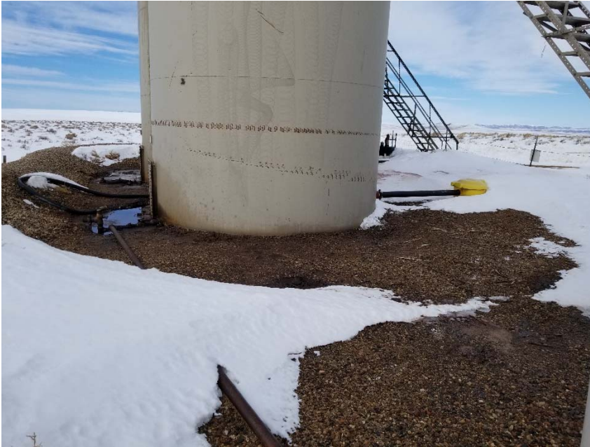
Photo 3. Stained soil and free product around base of tanks.
