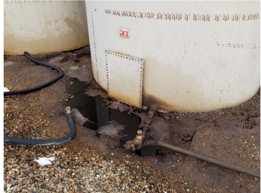
Photo 4. Stained soil and free product around base of tanks.
