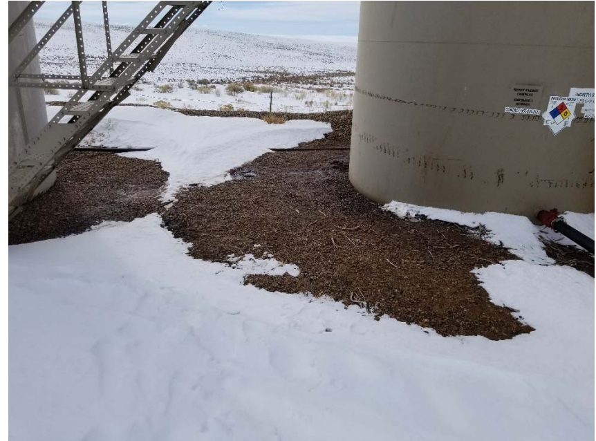
Photo 2. Stained soil and free product around base of tanks.
