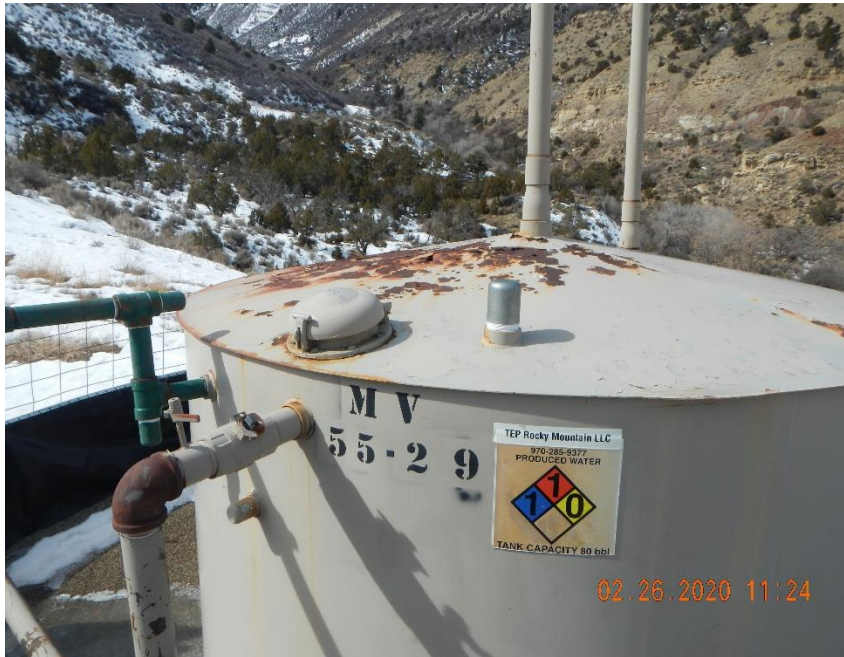
Top of produced water tank is rusted out.
