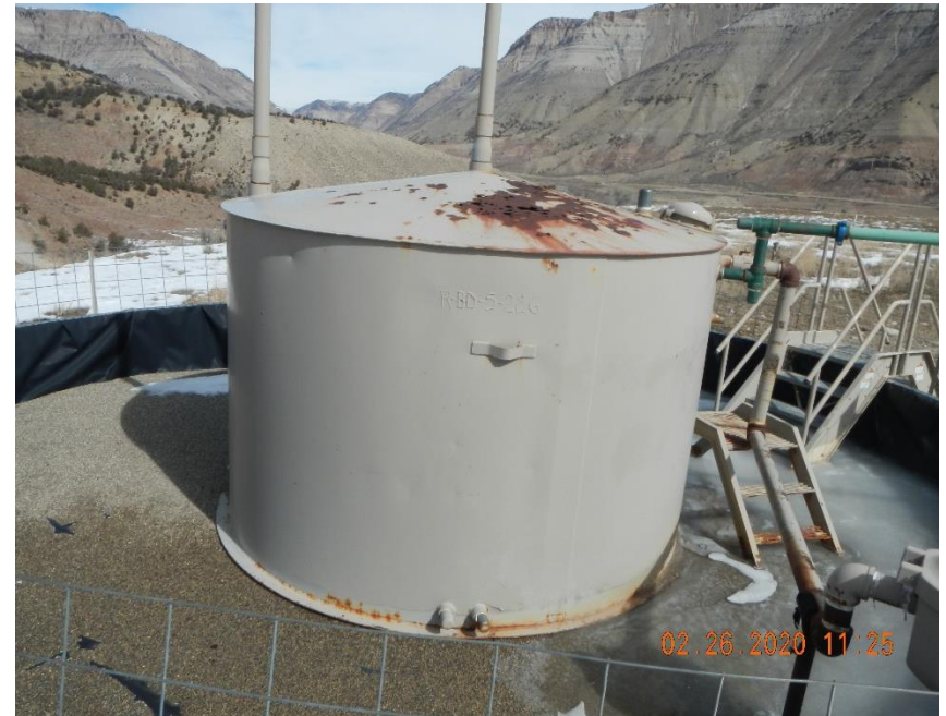
Top of produced water tank is rusted out.
