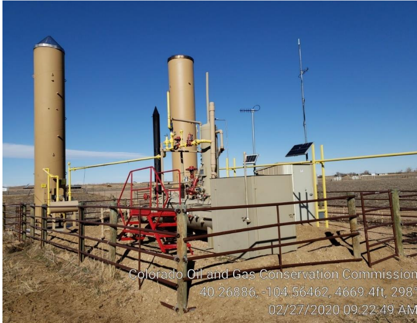
Photo #2 Separator, ECD's & Meter Run
