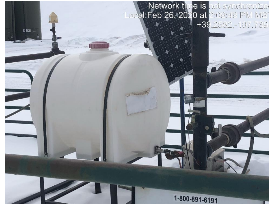
Photo #0653 Chemical tank label weathered and not legible.
