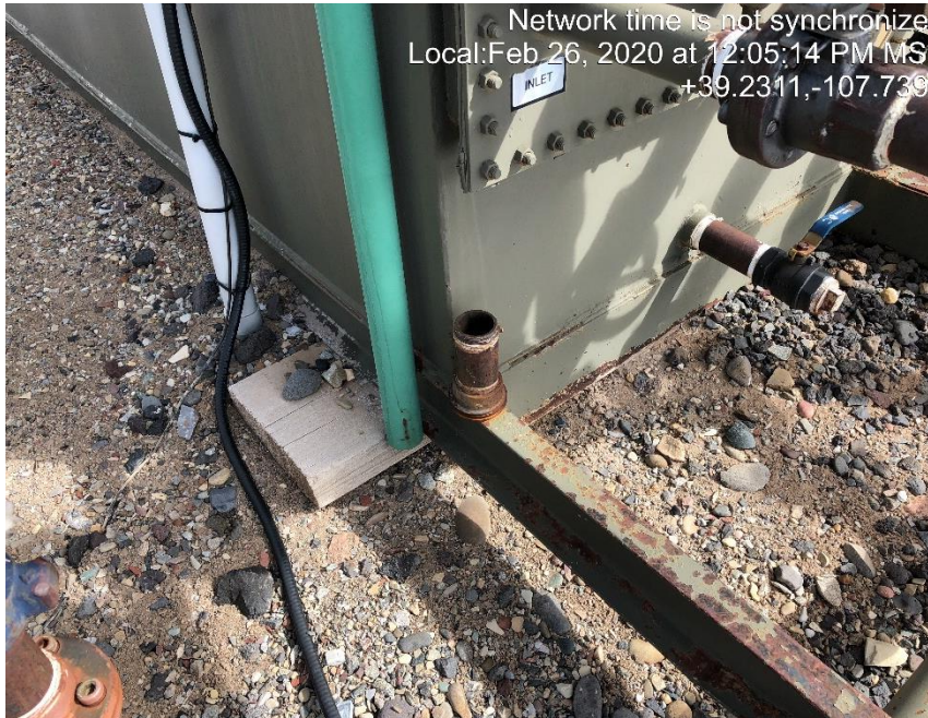
Photo #0644 unused thread half and nipple on separator.
