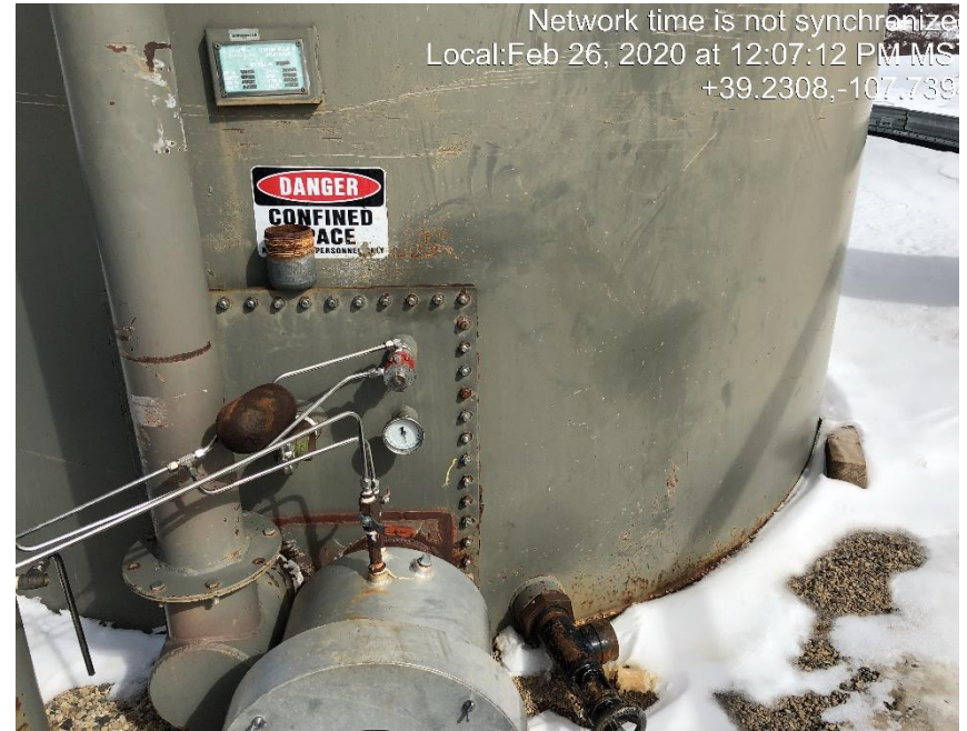
Photo #0645 unused bull plugs on tank burner.
