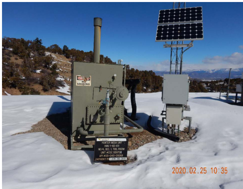
Photo #5 – Horizontal heated separator
