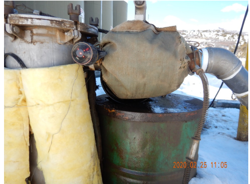
Photo #18 – Close up view of condensate accumulation on upper tank battery loadout equipment.
