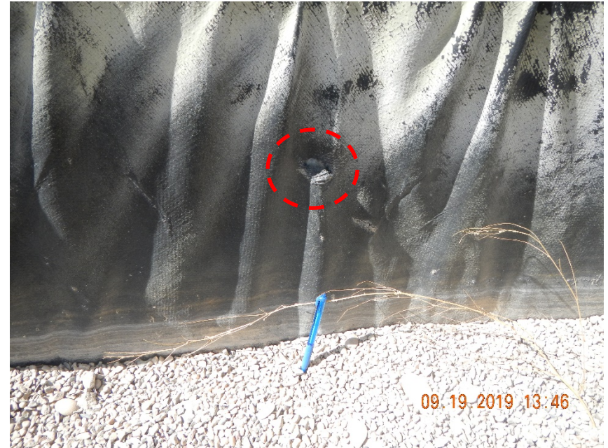
Photo #12 – Photo (#4) from previous Field Inspection Report (doc #699700034, photo dated 9/19/2019). Similarities in size and shape of hole as well as patterns in nearby paint suggest that this is the same location as previous photo.
