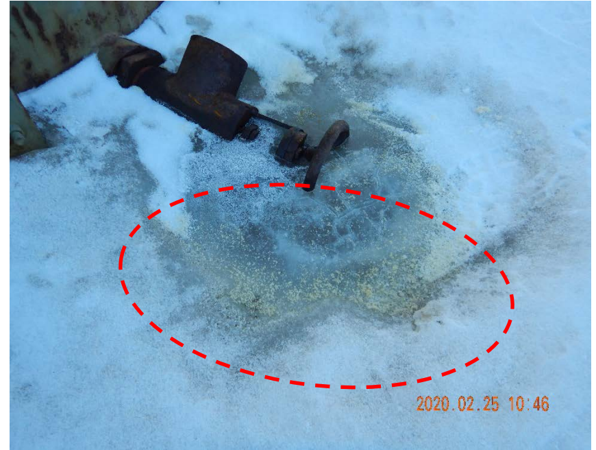
Photo #10 – Valve on north tank lacks bullplug, condensate staining observed in this location.
