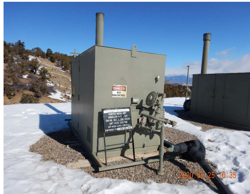
Photo #4 – Horizontal heated separator
