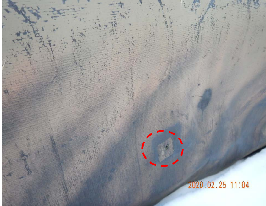
Photo #21 – Hole in upper tank battery liner appears to have been patched previously.
