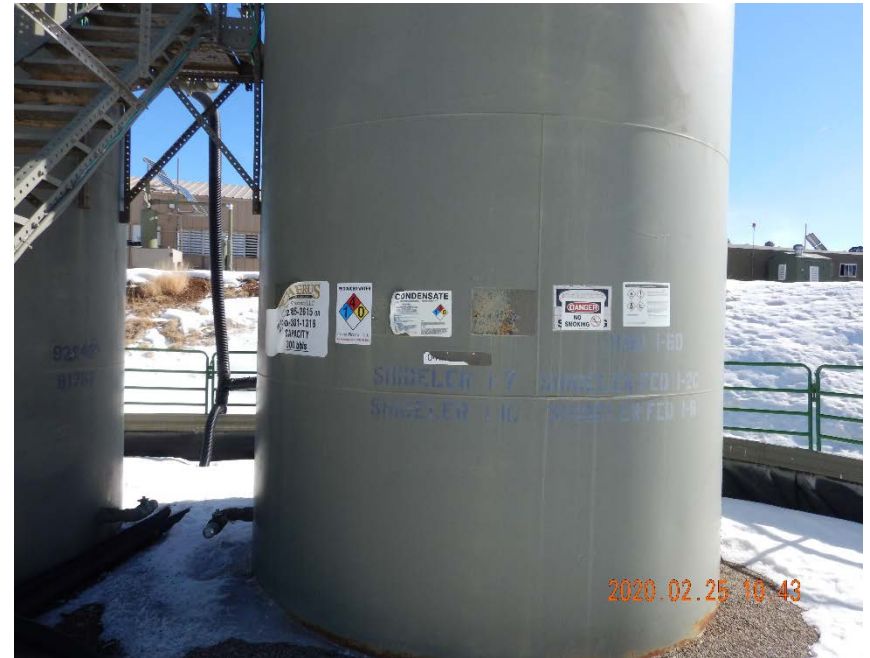
Photo #8 – Tank labels damaged at lower tank battery (south tank).
