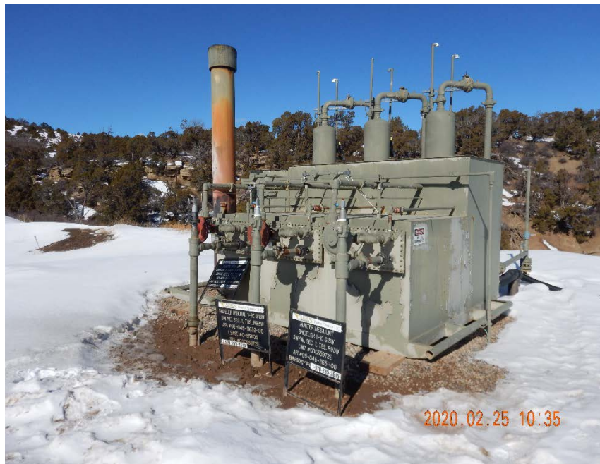
Photo #3 – Vertical heated separators.
