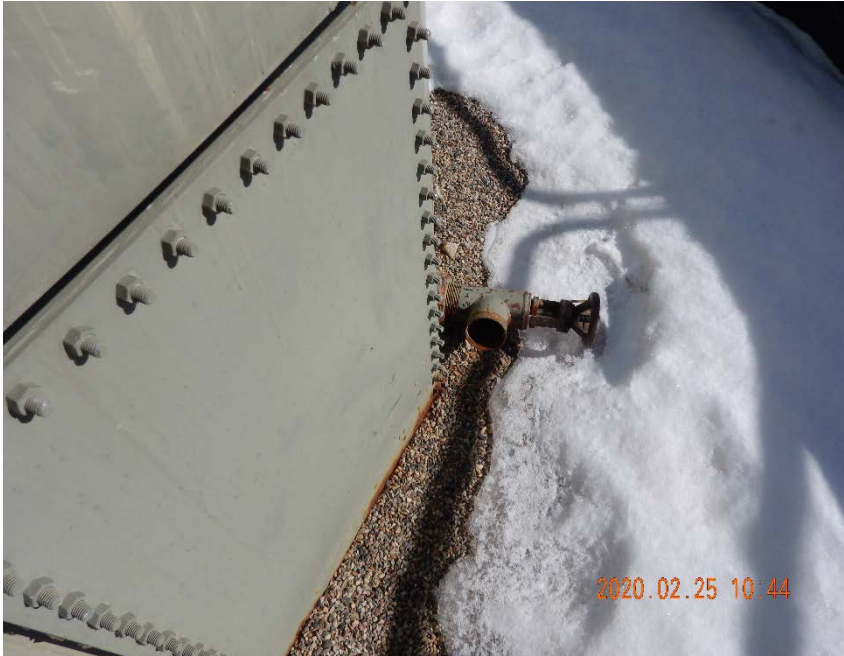
Photo #9 – Valve on south tank lacks bullplug.
