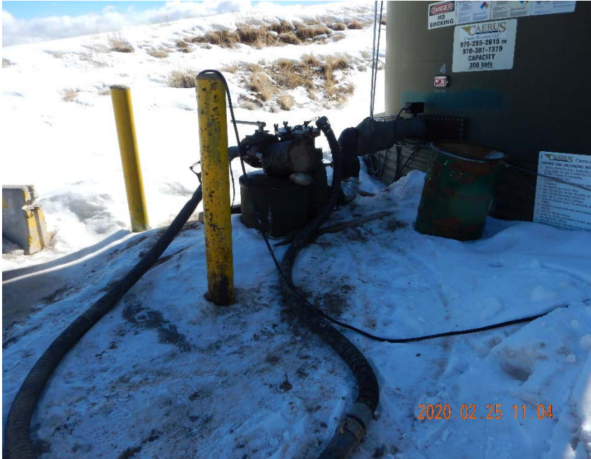
Photo #17 – View of upper tank battery loadout area. Note condensate staining on ice.
