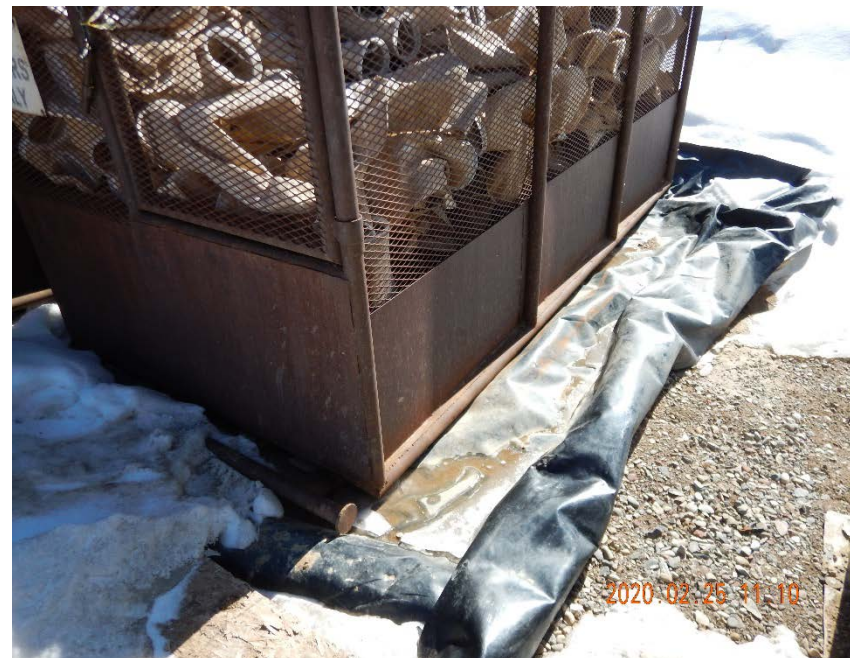
Photo #26 – Close up of liner beneath waste containers.
