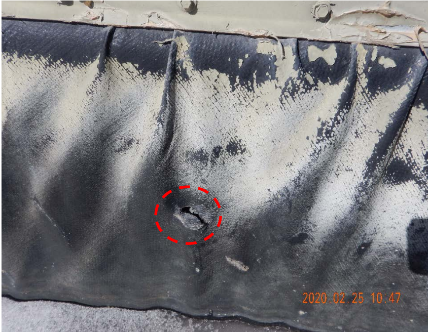
Photo #11 – Hole in lower tank battery liner noted in previous Field Inspection Report (doc #699700034).
