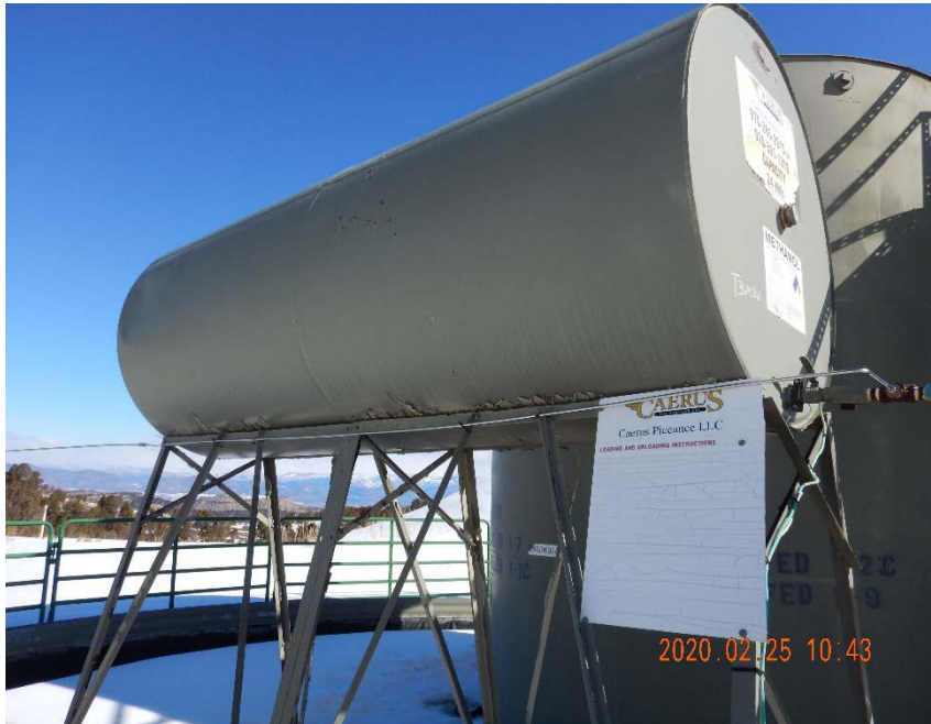
Photo #7 – 24 bbl methanol tank in lower tank battery, note faded sign.
