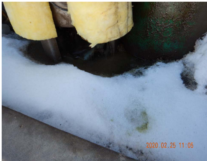
Photo #19 – Condensate accumulation in loadout area.
