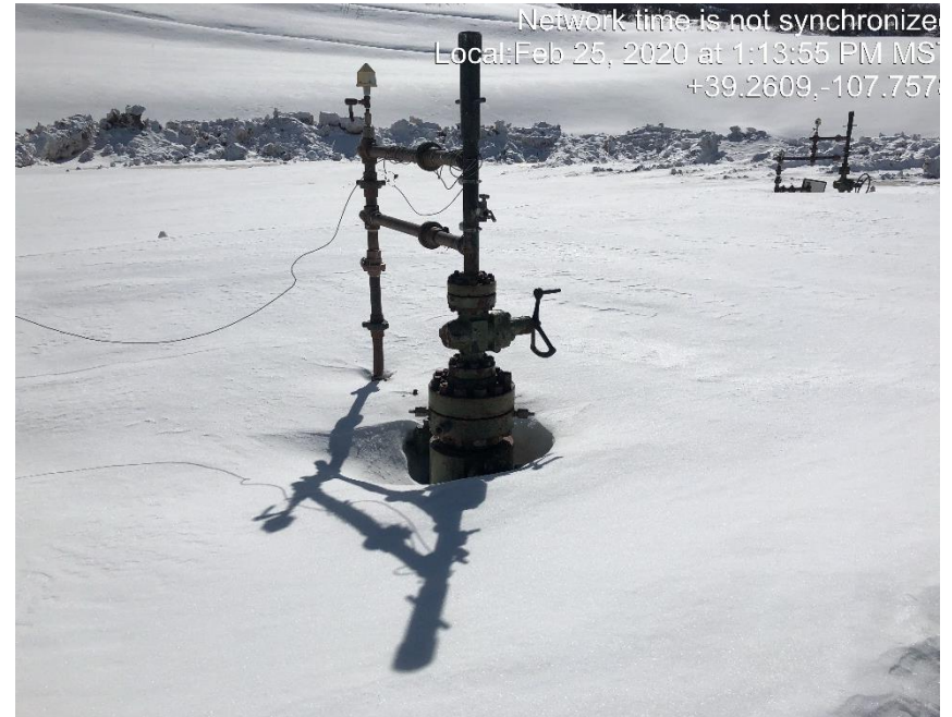
Photo #0638 Wellhead missing sign.
