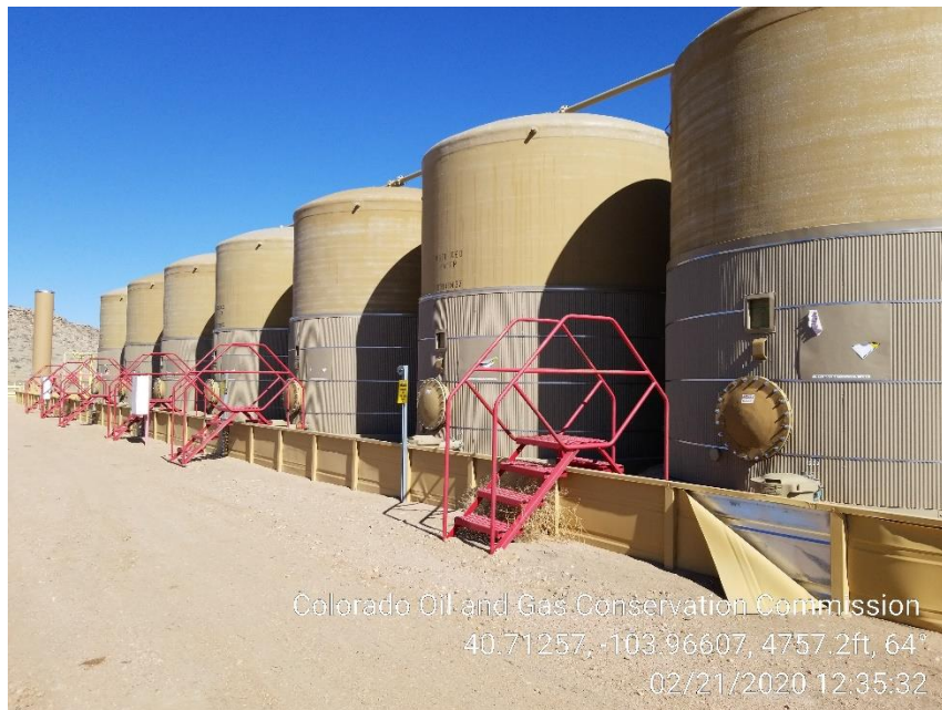
Photo 3 – Westside Water Tanks – Most Tanks are missing Content, Capacity and NFPA Labels
