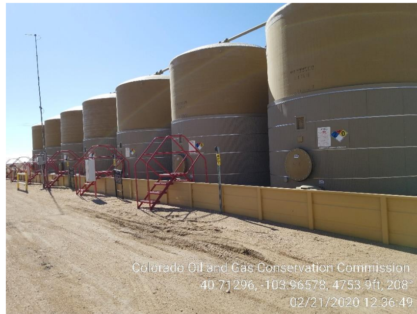
Photo 4 – Eastside Water Tanks – Most Tanks are missing Content, Capacity and NFPA Labels
