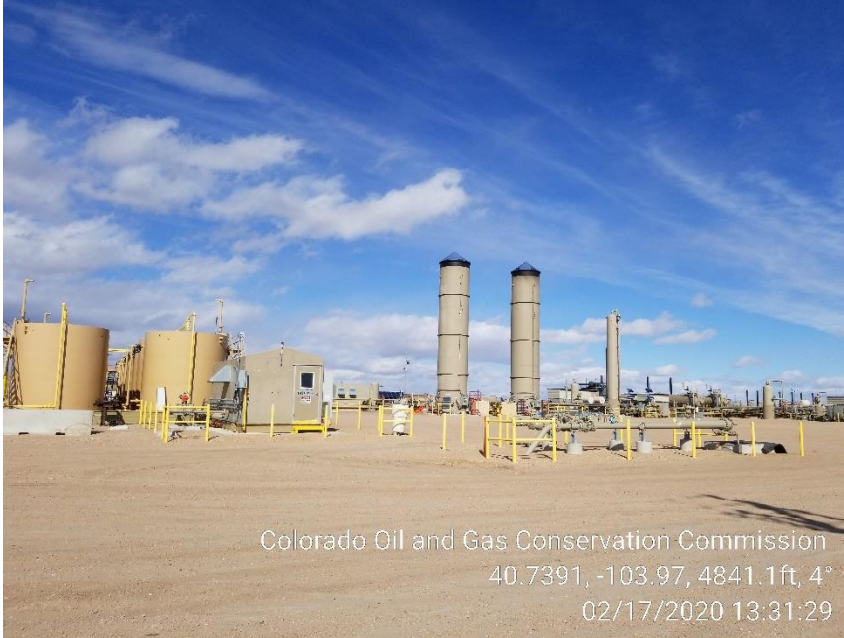
Photo 1 – Tank Battery
