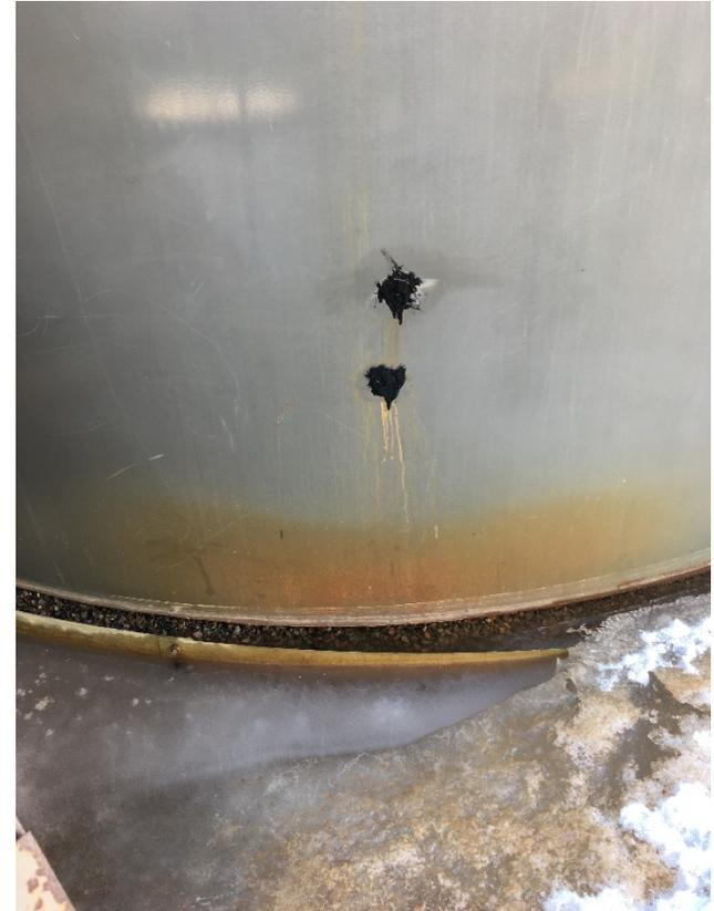
Produced water above ground storage tank, with repairs made in photo
