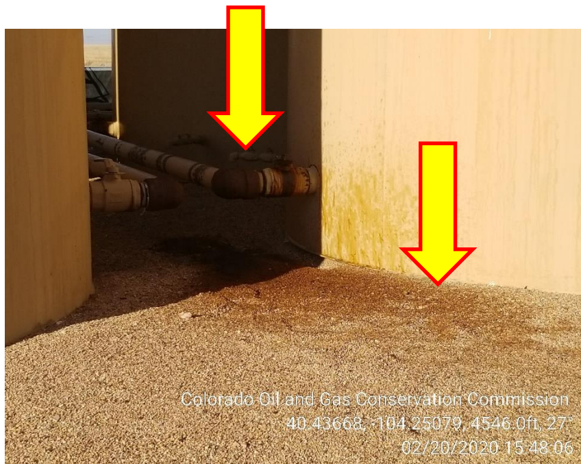
Photo 5 – Stained Soil at SE Tank inside Berm
