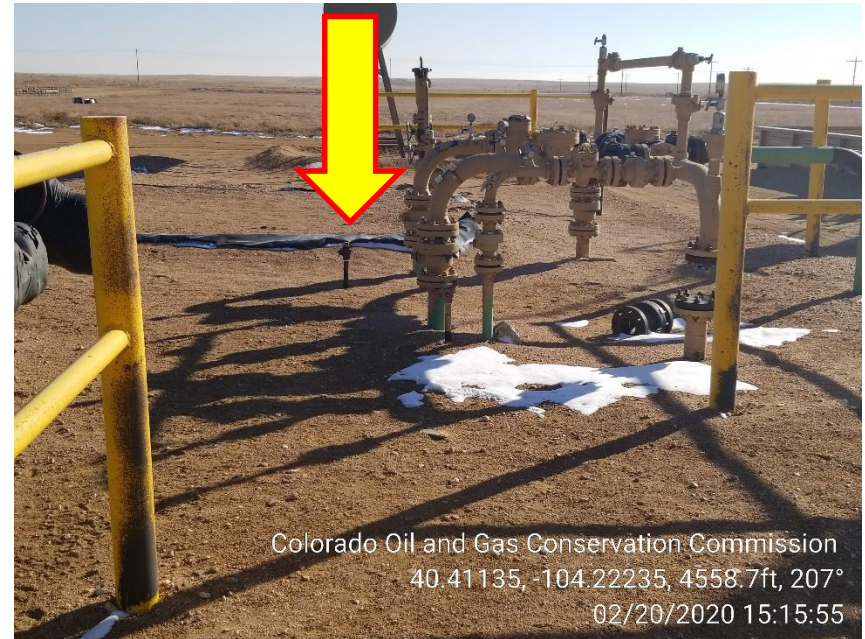
Photo 8 – Unmarked Riser West of Compressor
