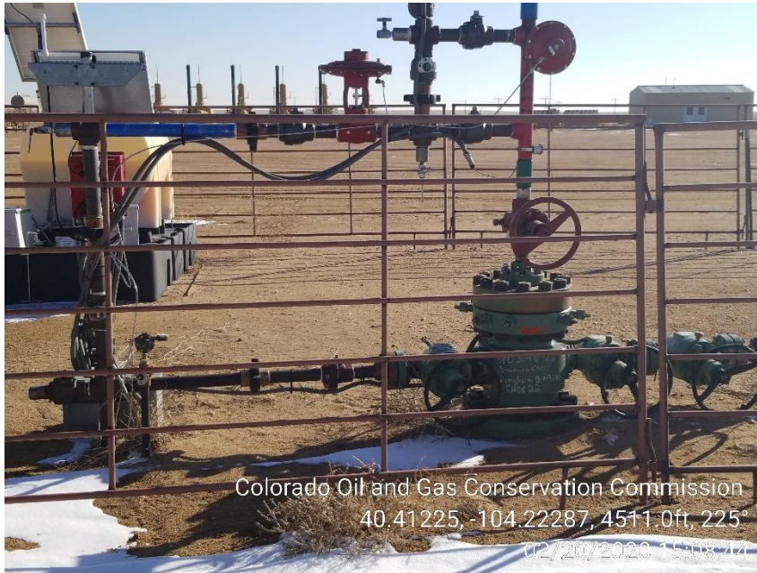
Photo 3 – D-X-9 Well missing Wellhead Sign
