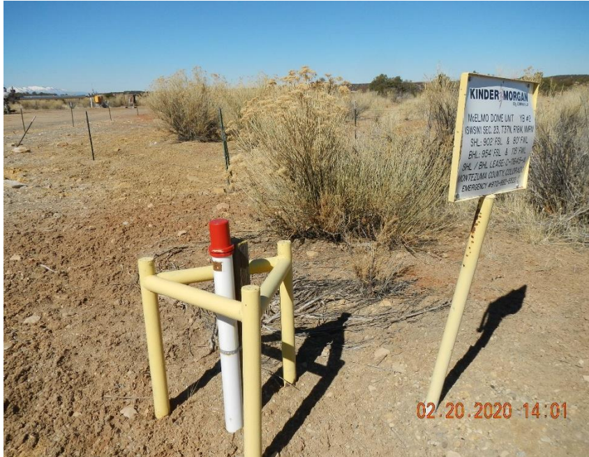
YB-2 location sign and cathodic protection test station.
