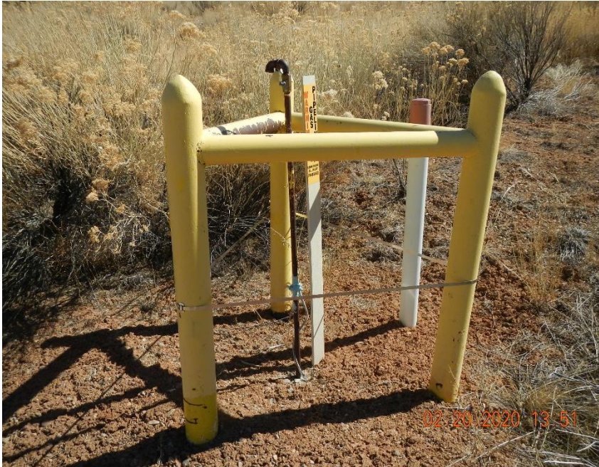
Flow line vent and cathodic protection standpipe.
