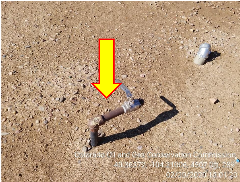
Photo 5 – Unmarked Risers on the Eastside of location
