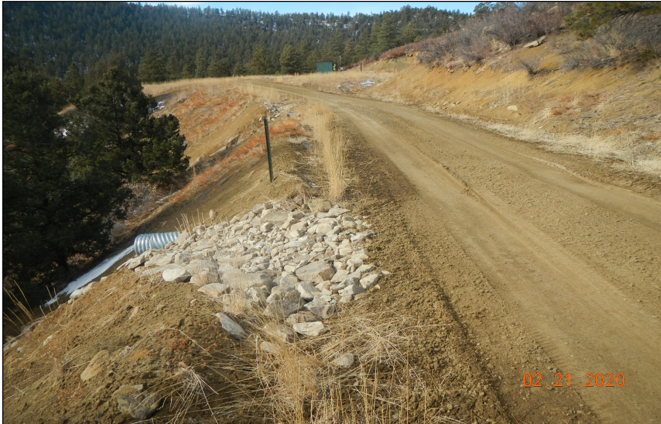
Photo 1. Facing southwest along the access road. Rock rip/rap has been installed near the culvert.
