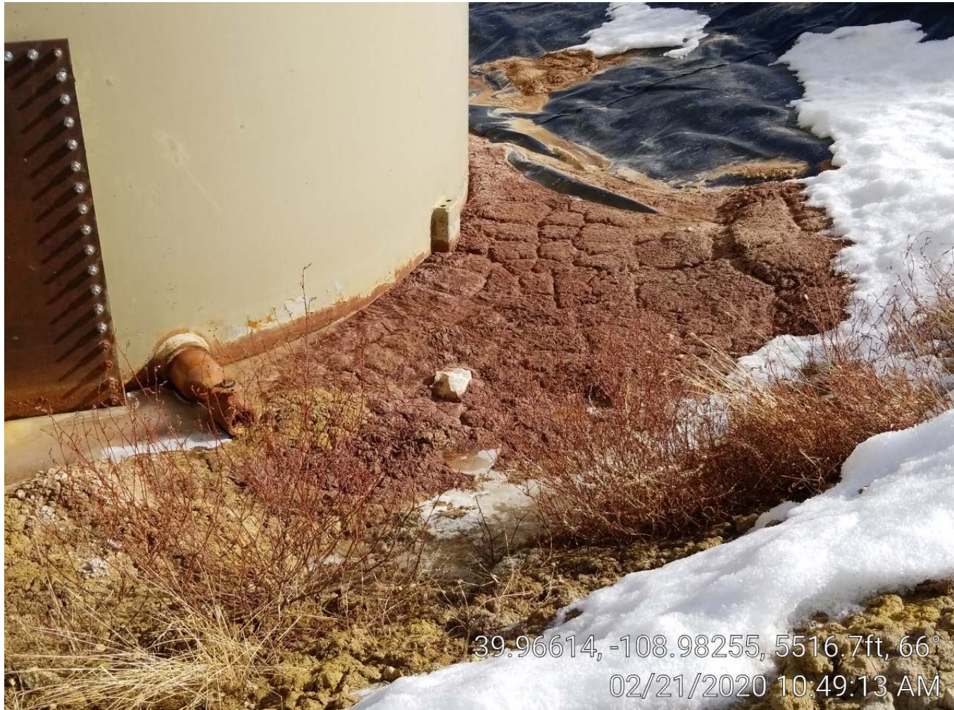
Photo 5. Stained soil next to tank.
