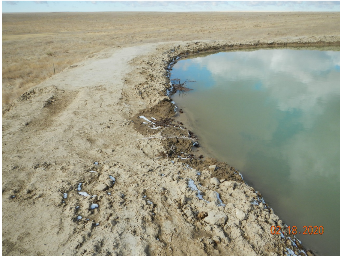
Photo # 8 – Pit 117462 not maintaining 2' of freeboard, wind caused waves could erode and breach pit berm
