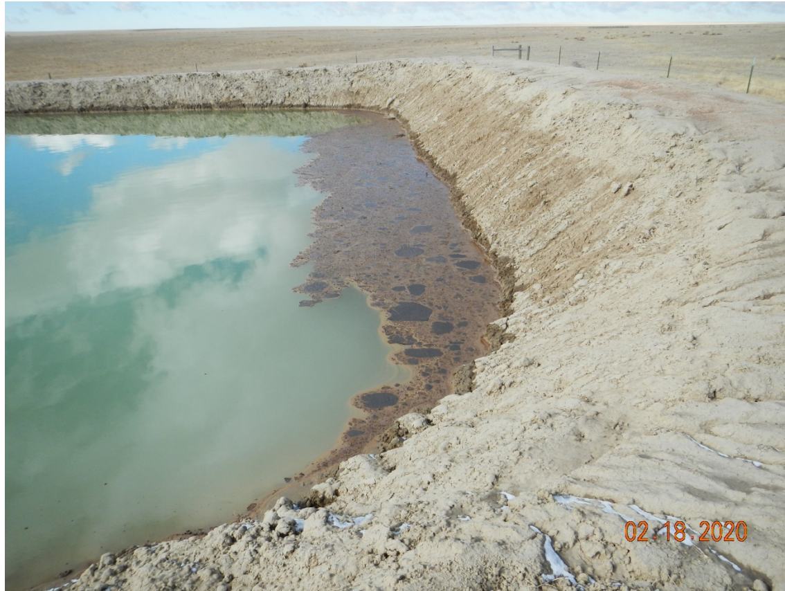
Photo # 5 – Pit 117462 not maintaining 2 feet of freeboard, oil accumulation on surface at north end due to wind direction
