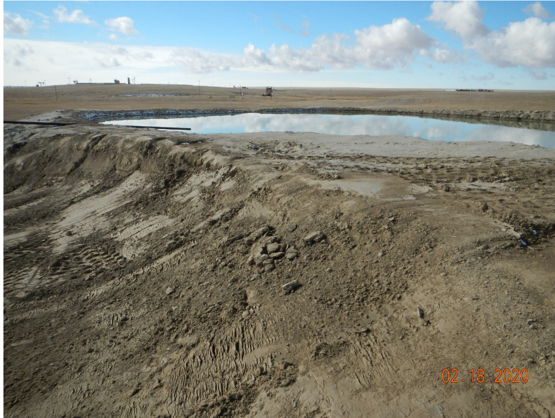
Photo # 4 – Pit 117462 not maintaining 2 feet of freeboard, probably 4" of freeboard. Spill 465823 and Rem 14588 related to this pit
