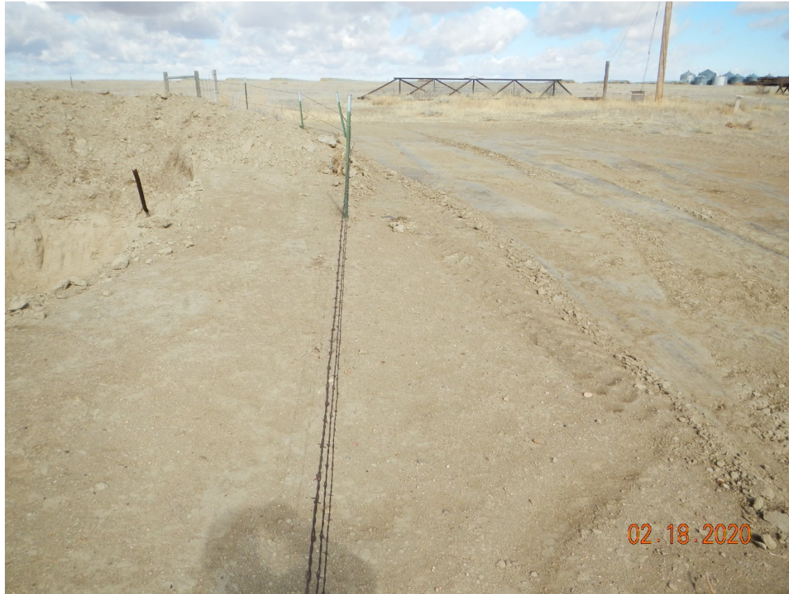
Photo # 2 – Oily soil stockpile has been removed, former oil skim pit cage remains on location
