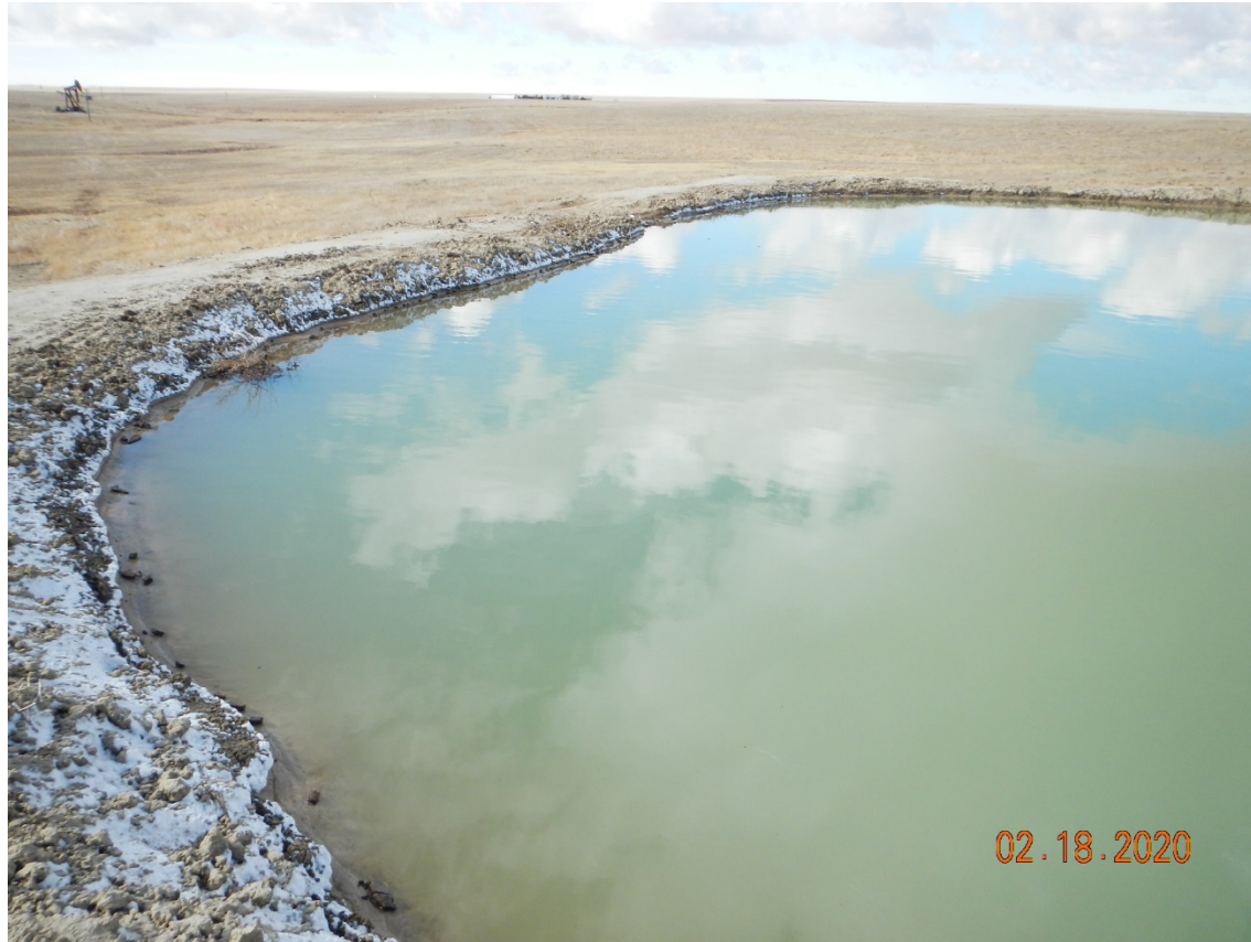
Photo # 6 – Pit 117462 not maintaining 2 feet of freeboard, view southwest
