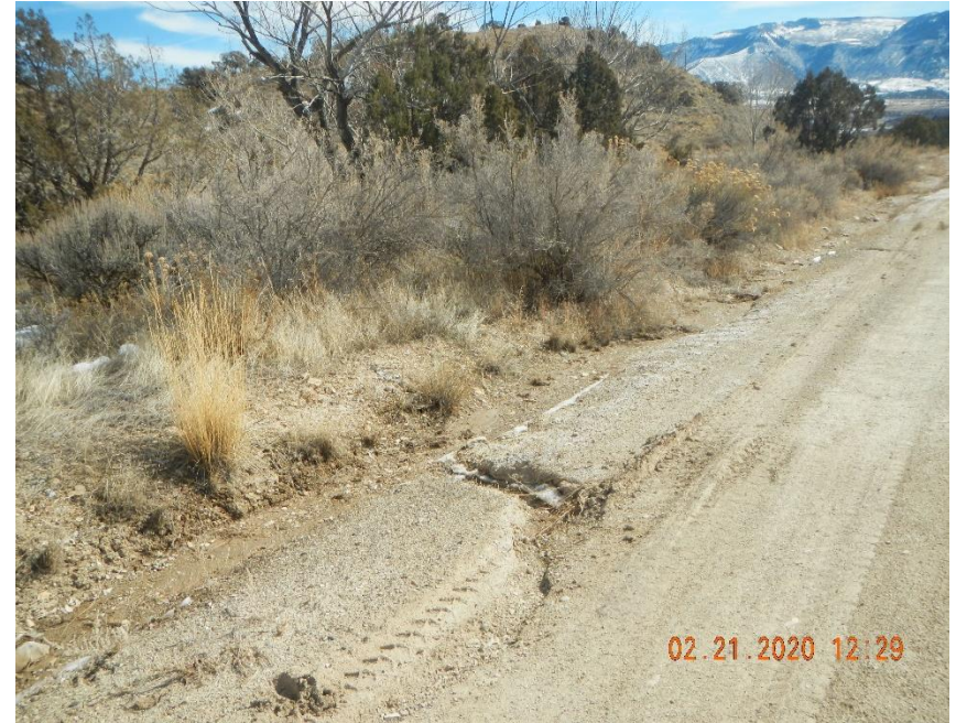
Ditch along access road needs maintained.
