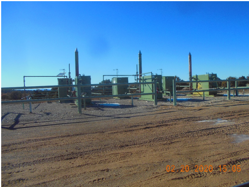
Separators and Meter housings with signs
