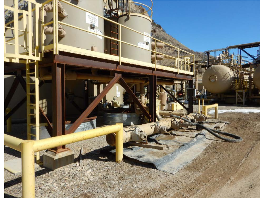
Photo #10 – Truck loadout manifold with hose located on south side of 15,000 bbl produced water/condensate AST.
