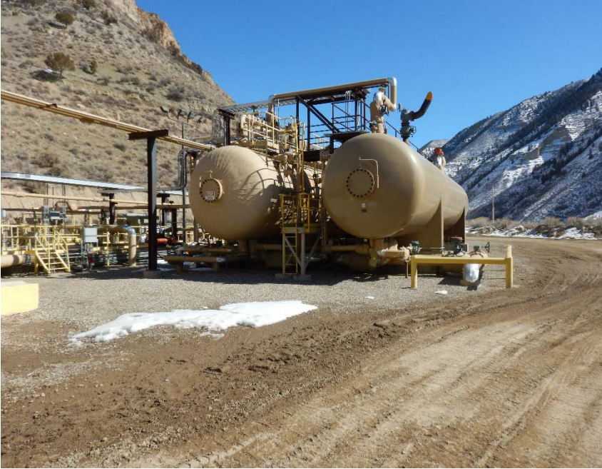
Photo #11 – Horizontal separators located east of 15,000 bbl produced water/condensate AST.
