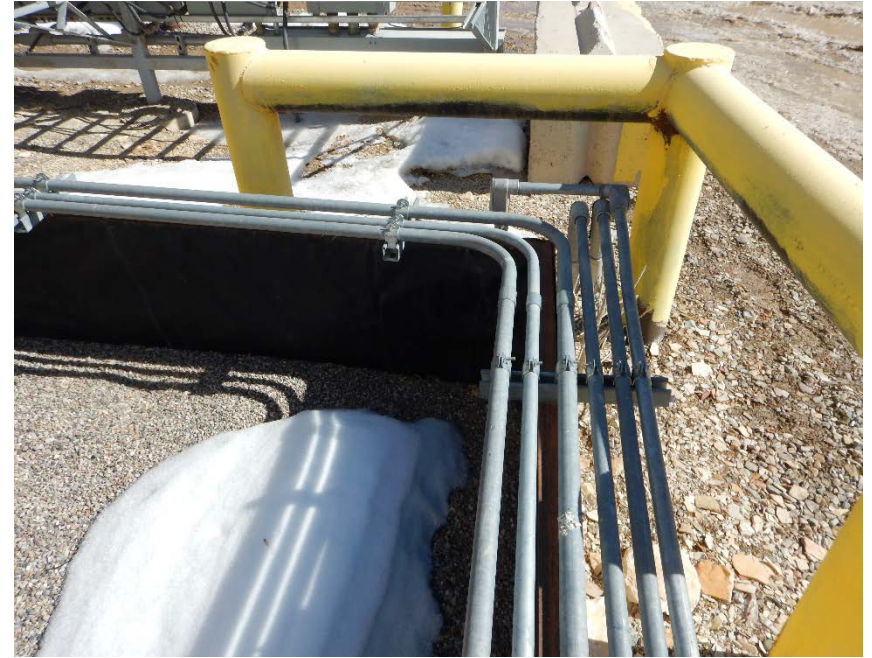
Photo #14 – View of southeast corner of secondary containment for upper condensate tank battery in “white tank” area. The secondary containment liner in this area had been repaired in response to previous FIR #698100063.
