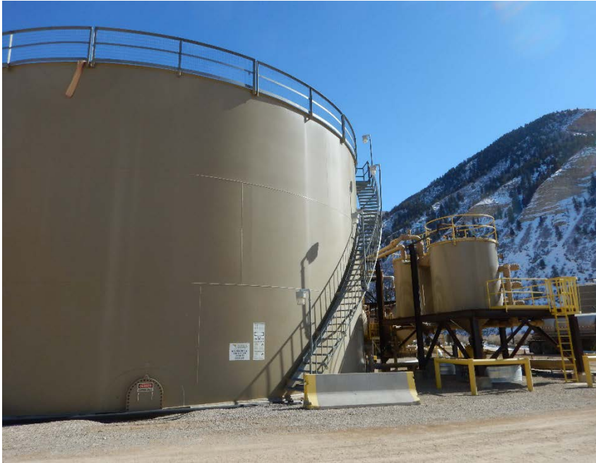
Photo #9 – View of 15,000 bbl produced water/condensate AST and two 110 bbl ASTs in “white tank” area, looking east.
