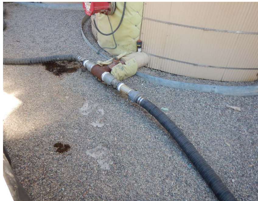
Photo #6 – Localized accumulation of oily waste beneath hose fittings on west side of tank battery.
