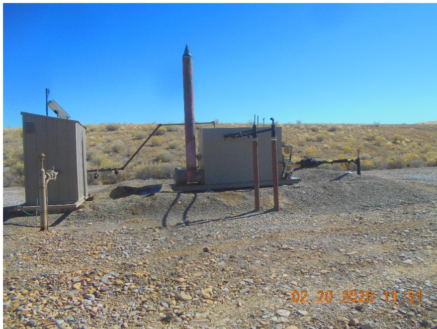
Separator and Meter housing
