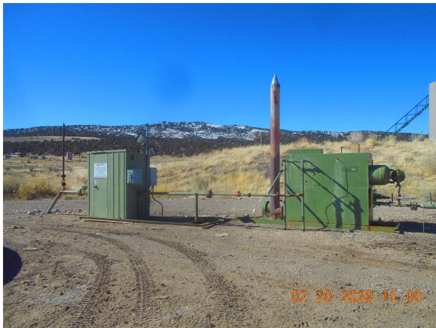
Meter housing with sign and Separator
