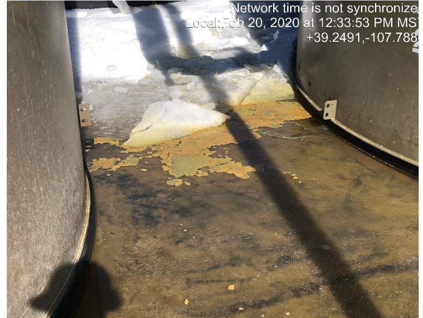
Photo #0615 Multiple places with paraffin and oily fluids in tank containment.
