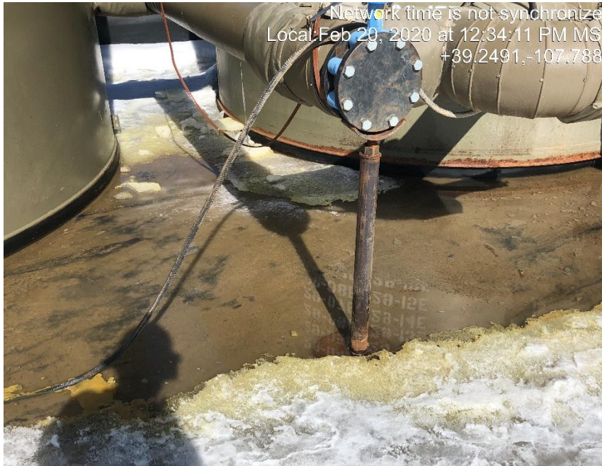
Photo #0616 Multiple places with paraffin and oily fluids in tank containment.
