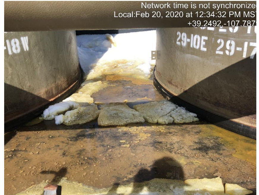
Photo #0617 Multiple places with paraffin and oily fluids in tank containment.
