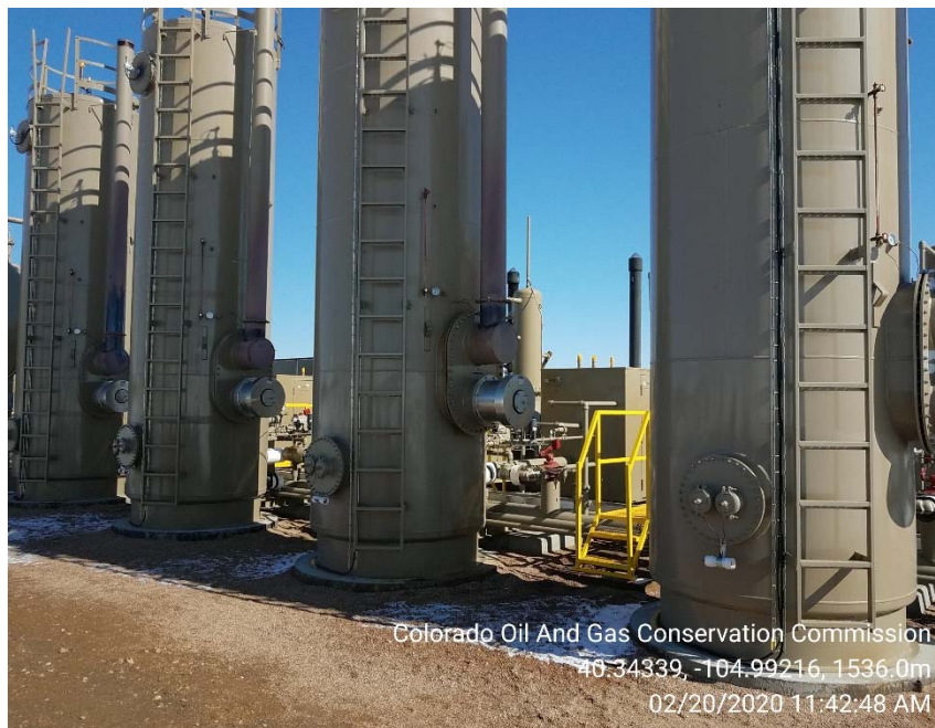
Vertical heater treater placards and berm
