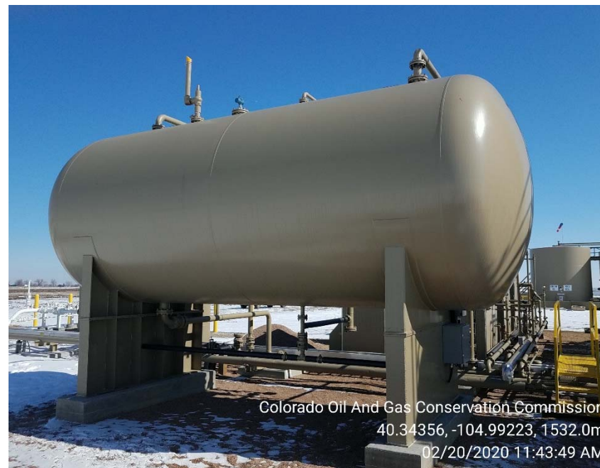
Oil knockout placards and berm
