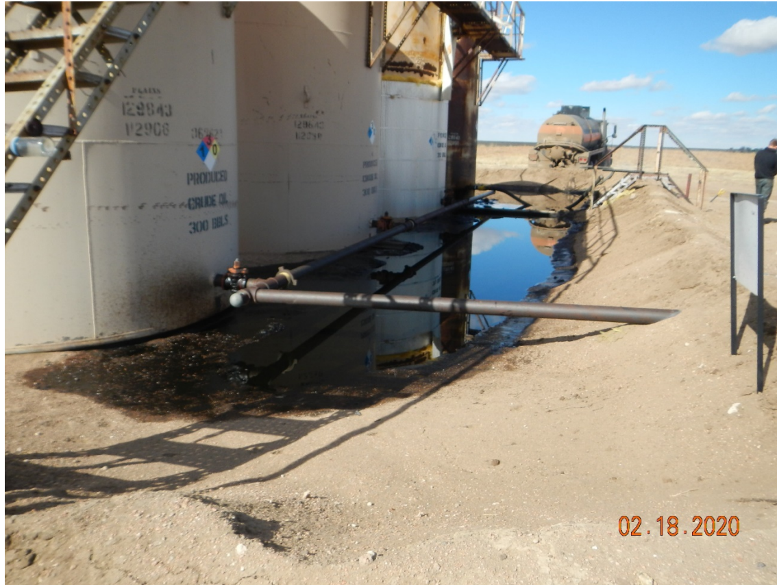
Photo # 2 – View north along east side of tank battery. Vacuum truck removing accumulated oil
