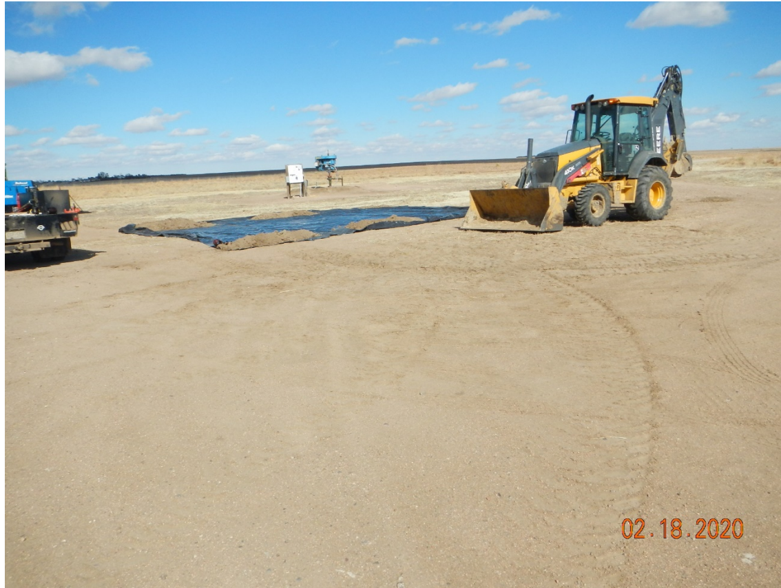
Photo # 4 – View northeast at plastic staged for impacted soil stockpile
