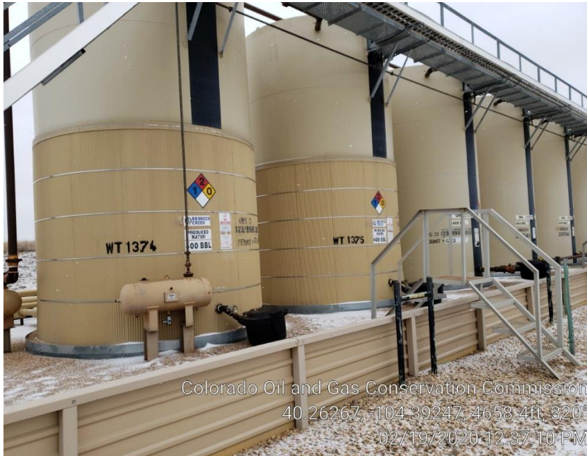
Photo #7 Capacity & Placards "NFPA" Are legible on water tanks.
