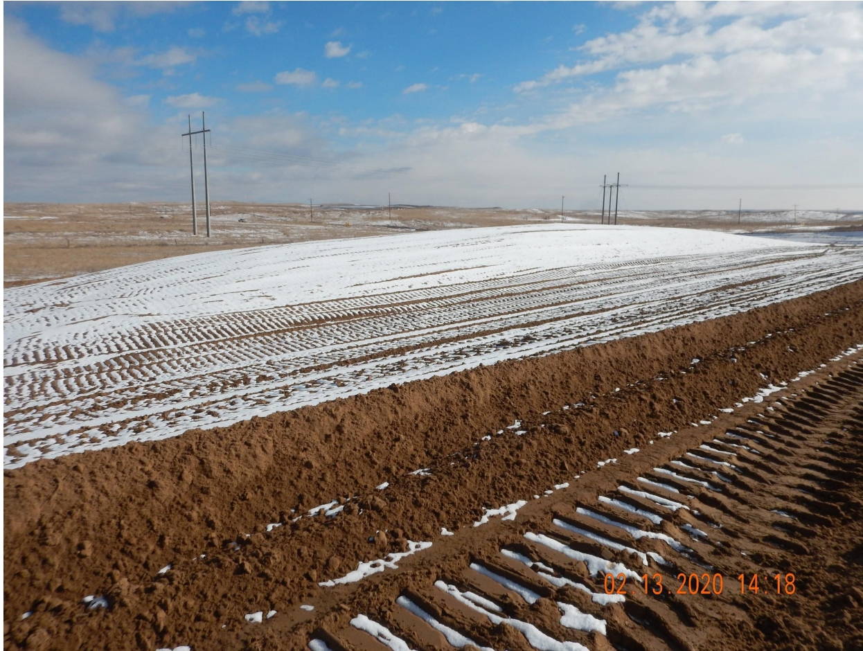
Photo 9. Photo taken from the eastern perimeter of location, facing Southeast. Photo illustrates the topsoil stockpile which has been temporarily stabilized with equipment tracking.
