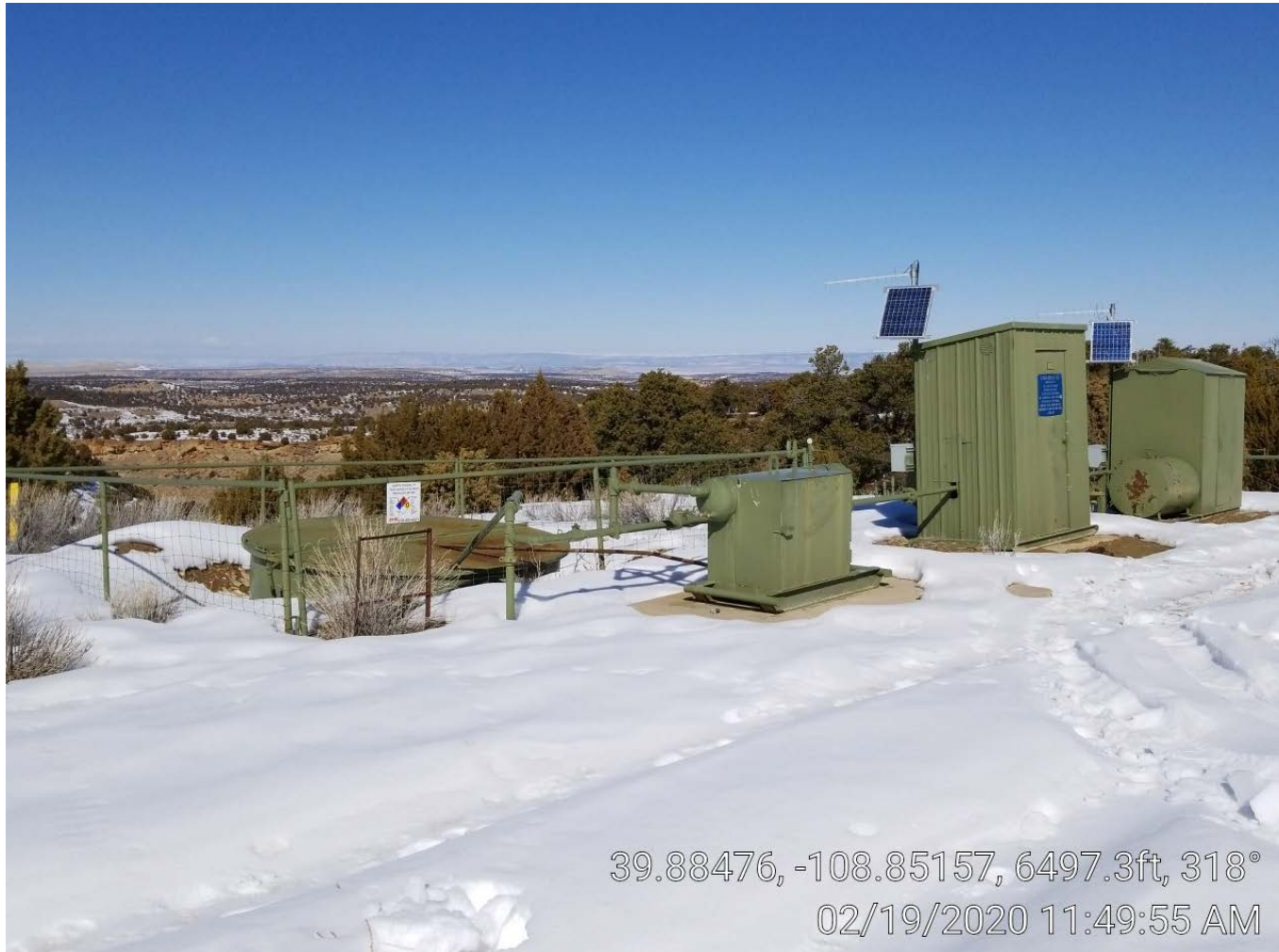
Photo 2. Tank & meter buildings.
