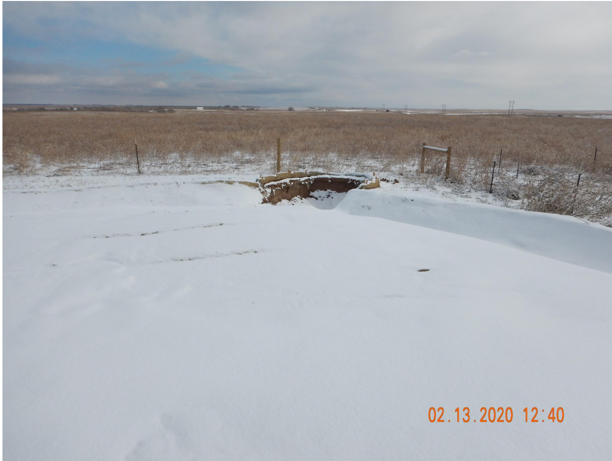
Photo 1. Photo taken from the southeastern perimeter of location, facing East. Photo illustrates Operator appears to have installed a sediment trap. Per good engineering practices, a sediment trap should have side slopes of 2:1 or flatter and should have a stabilized outlet. The above sediment trap has vertical side slopes that are susceptible to sloughing and no stabilized outlet. Wattles are not intended to filter stormwater but rather pool stormwater.
