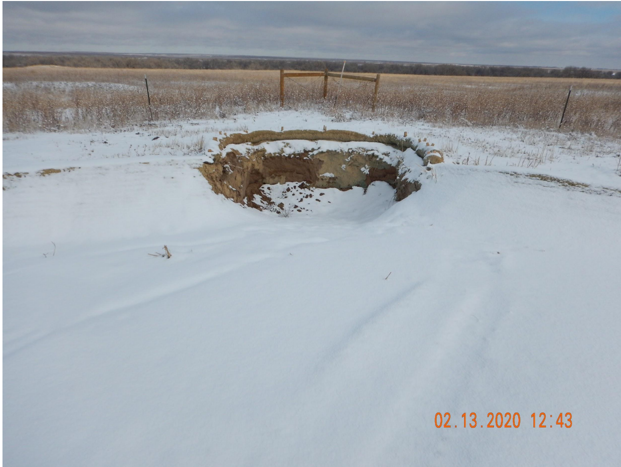
Photo 3. Photo taken from the northeastern perimeter of location, facing East. See comments under Photo 1. Note, with the vertical side slopes, it appears sloughing is already evident. It appears the Operator has also applied hydromulch but that did not prevent sloughing.
