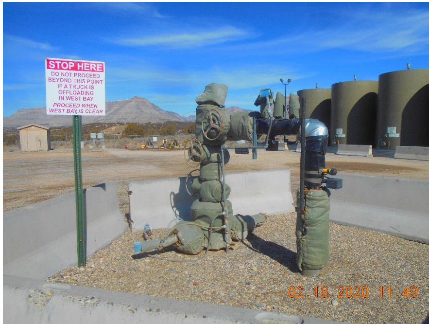
Injection wellhead with cement barricades
