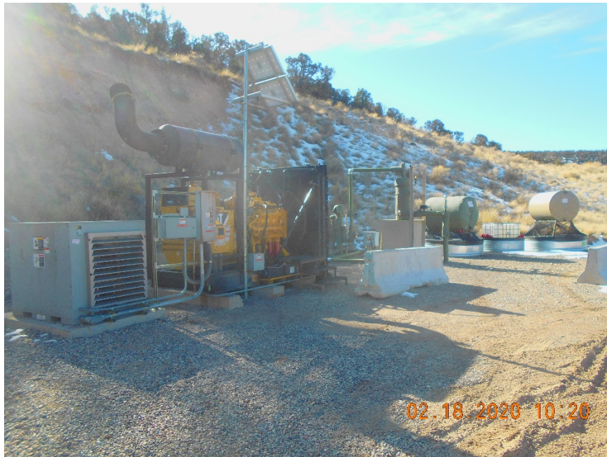
Generator and Stored chemicals with secondary containment
