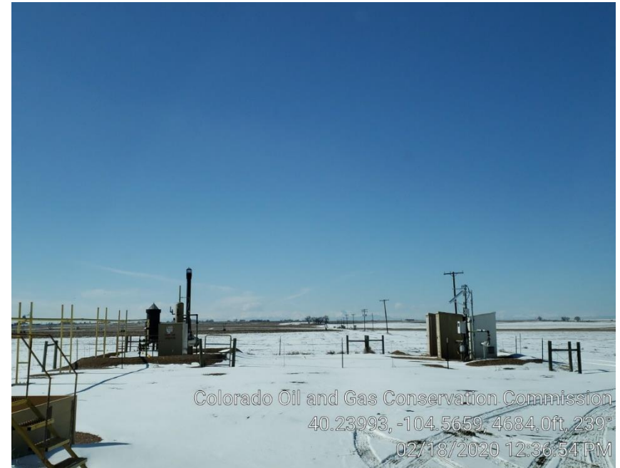
Photo #2 Separator, ECD & Meter Runs
