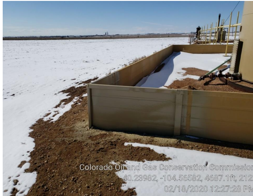
Photo #3 Fixed Secondary containment wall
