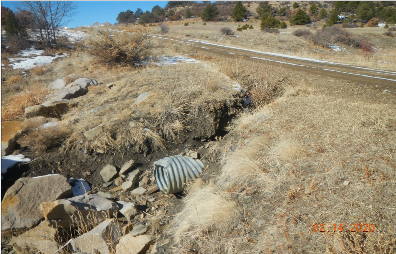
Photo 1. Stormwater drainage from the main road is causing erosion near the culvert at Lat/Long:37.13600,-104.83819.
