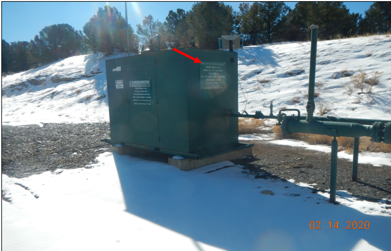
Photo 3. Well sign is installed at meter shed. Old operator sign (red arrow) should be removed.
