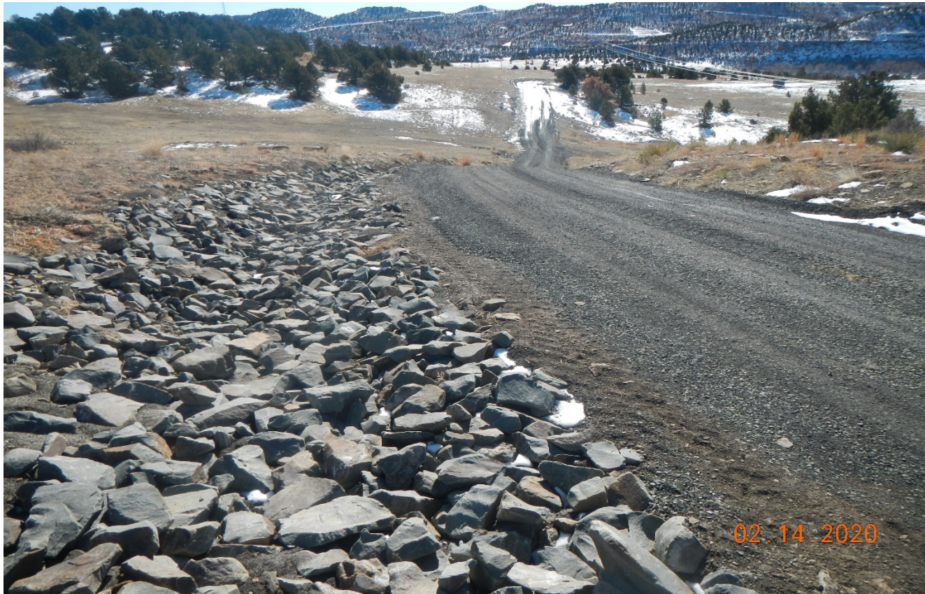
Photo 2. Facing southeast along the access road. Rock rip/rap has been placed along the side and gravel on the access road.
