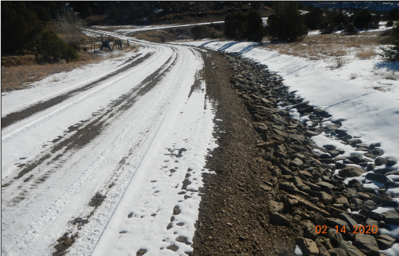
Photo 1. Facing east along side of the main access road. Erosion repairs have been made since previous inspection.
