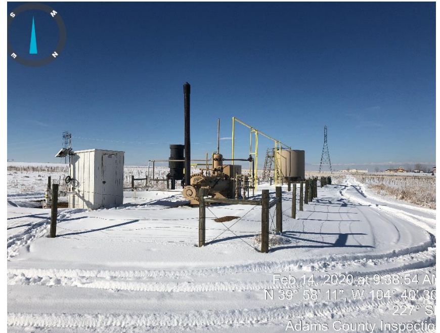
Photo #2 ECD, separator and meter run
