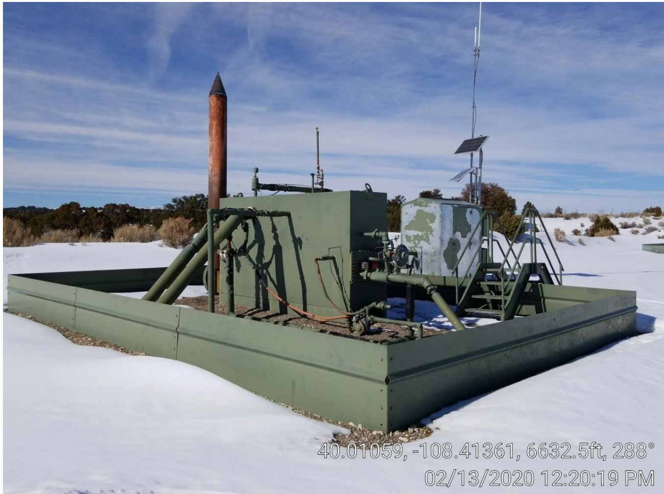
Photo 3. Separator & meter building.
