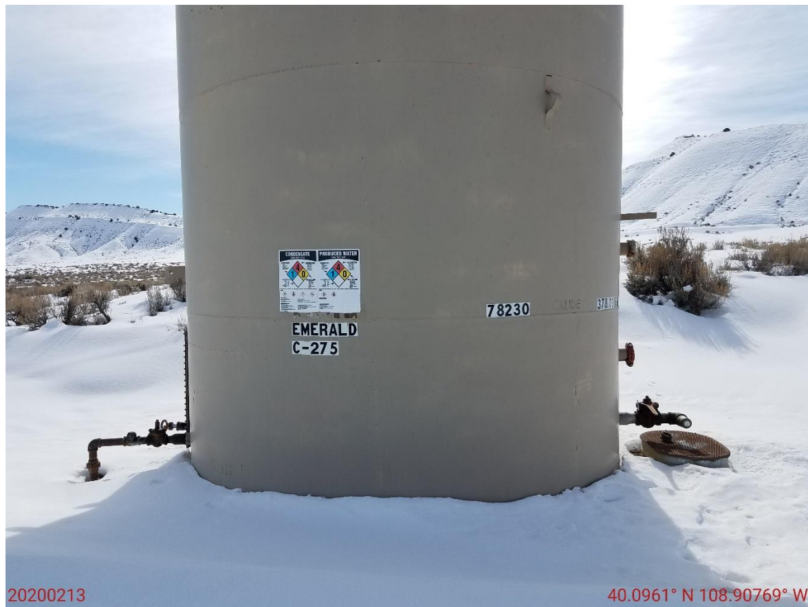
Photo 22: Photo taken from that south end of the Emerald #275 well Location, facing south. Photo shows current active produced water tank on the Location. Label indicates capacity @378.03 bbl. Signage on tank matches with signage on stored tank in photo #14; It appears the tank in photo 14 was replaced with this tank, was then stored on site rather than removed.
