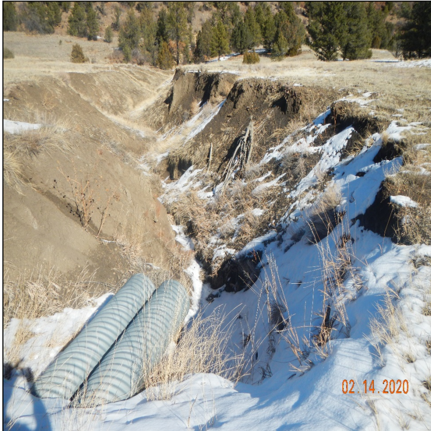
Photo 3. The stormwater outlet from this culvert is contributing to erosion of this gully. Lat/Long:37.14492,-104.86948.
