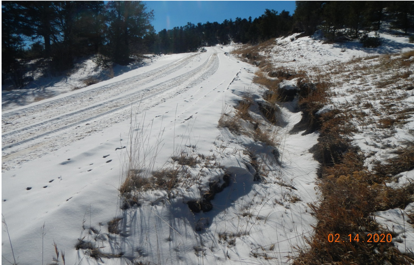
Photo 5. There a deep erosion channel along the access road at Lat/Long:37.14899,-104.87705.
