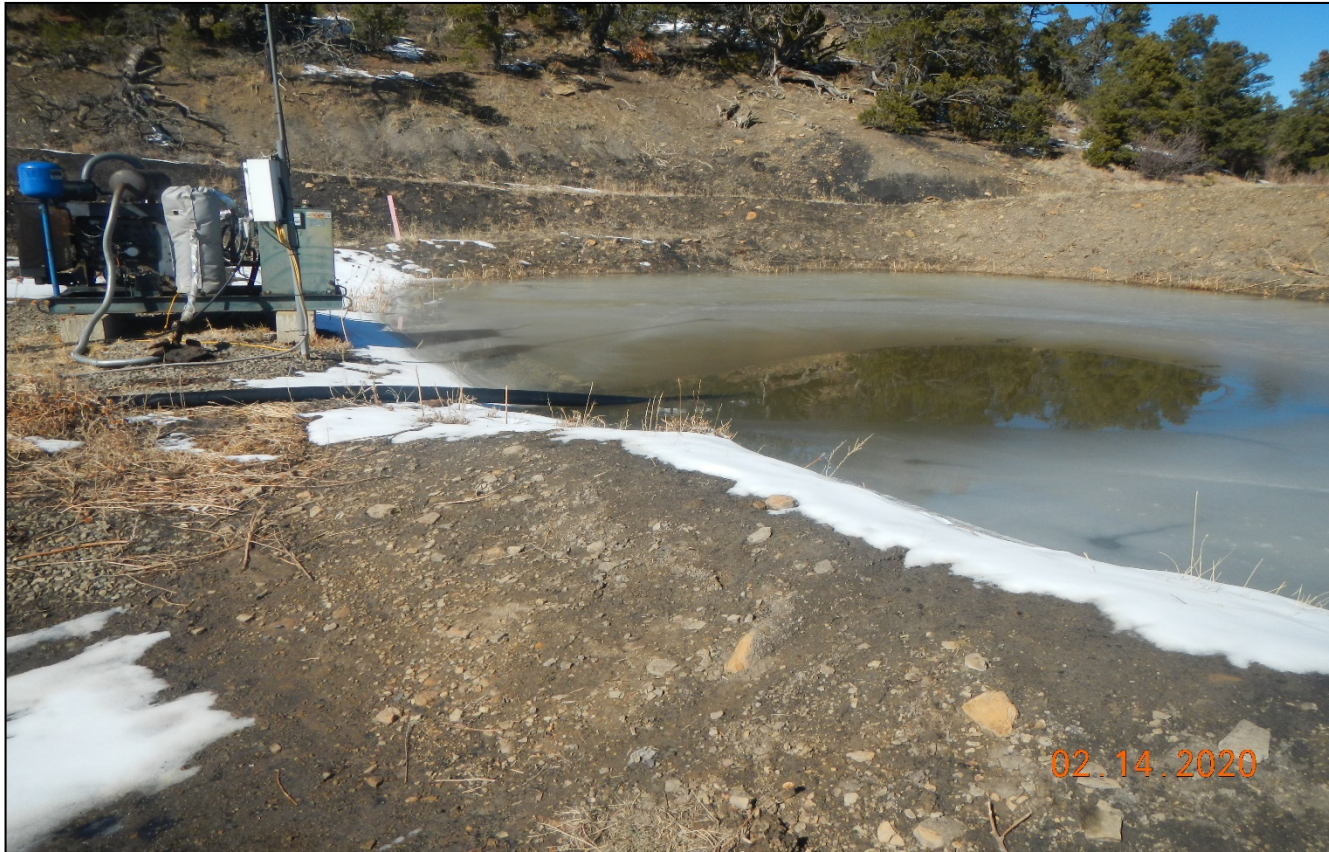
Photo 7. The water level at the pit is approaching 2 ft. freeboard and needs to be lowered.
