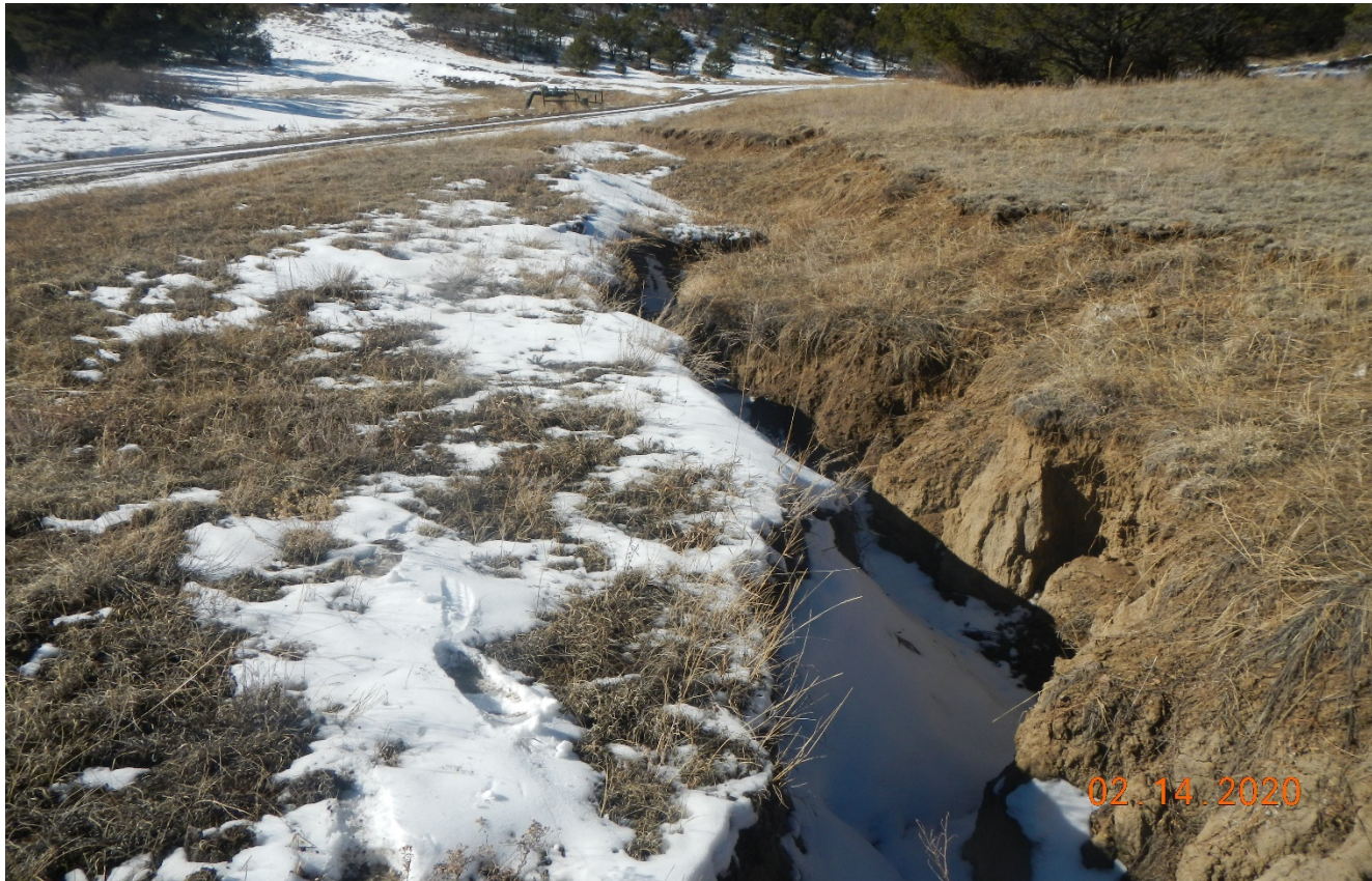
Photo 1. There a deep erosion channel along the main access road from stormwater runoff from the road at Lat/Long:37.14482,-104.86800. This area needs to be repaired and reclaimed.
