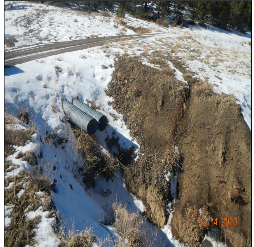
Photo 3. The stormwater outlet from this culvert is contributing to erosion of this gully. Lat/Long:37.14492,-104.86948.
