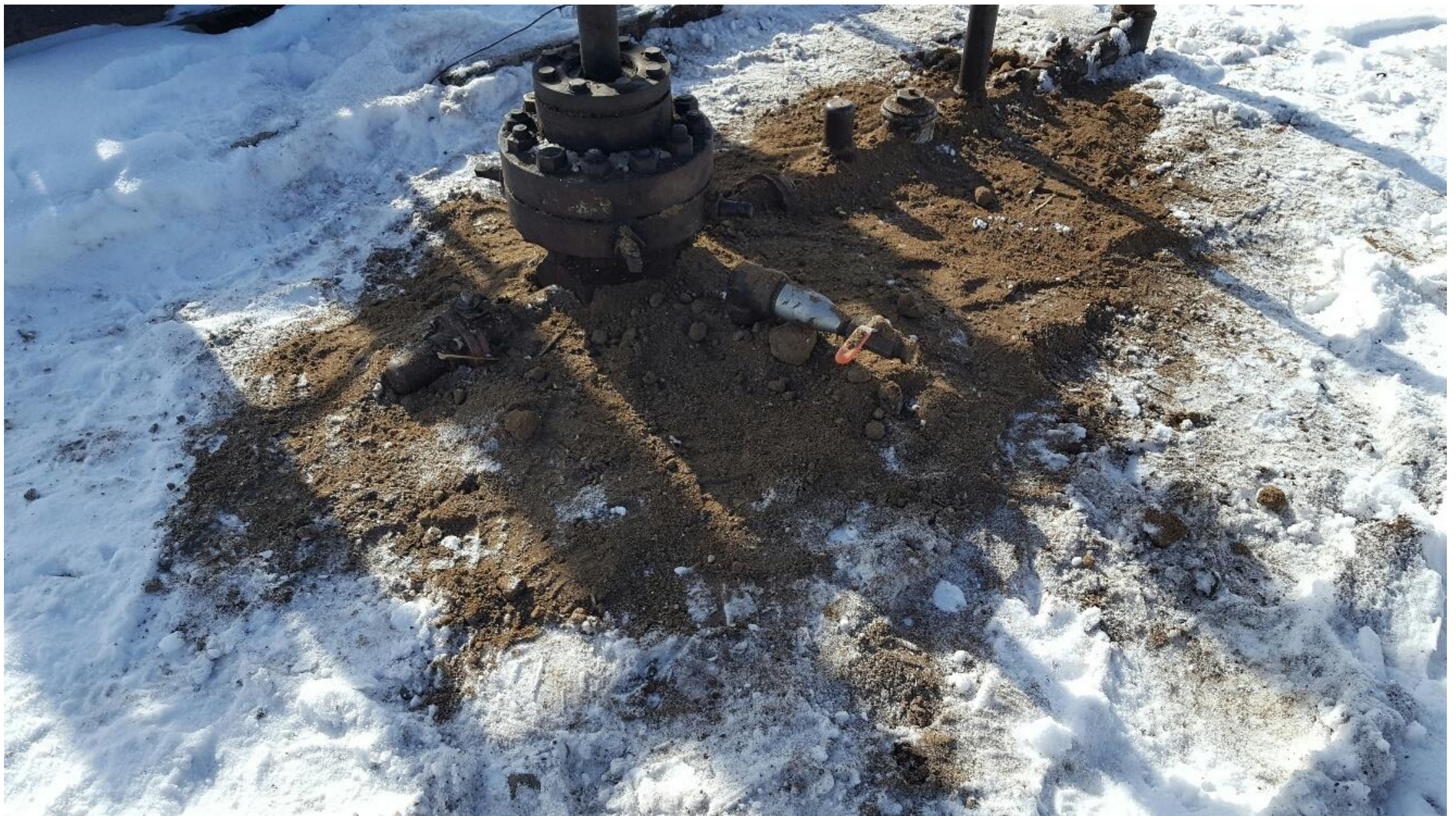
Figure #1 Stained soil has been removed.
