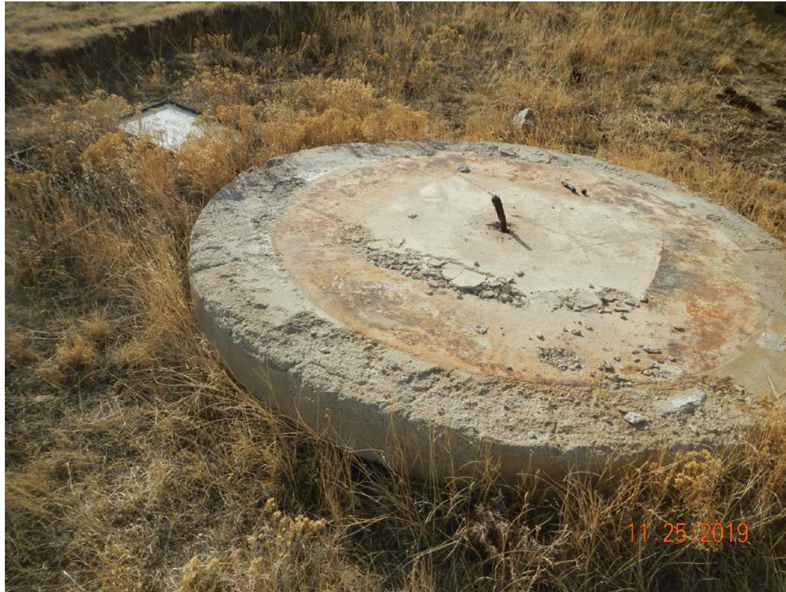
Photo # 2 – Concrete separator foundation, requires removal and proper disposal
