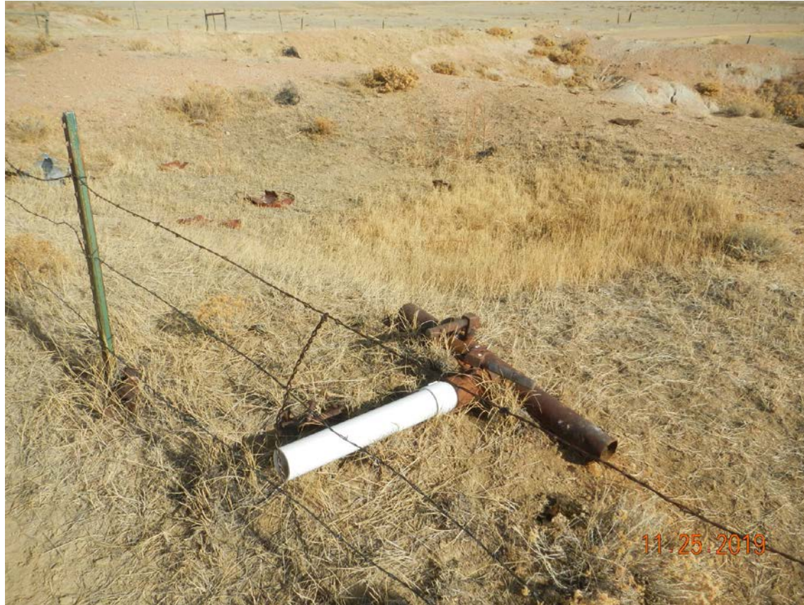
Photo # 4 – Risers require proper abandonment. Located on west side of pit ID 107649.
