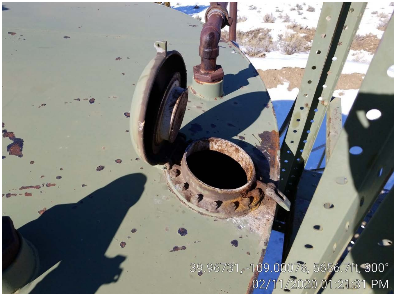
Photo 6. Open hatch on water tank.
