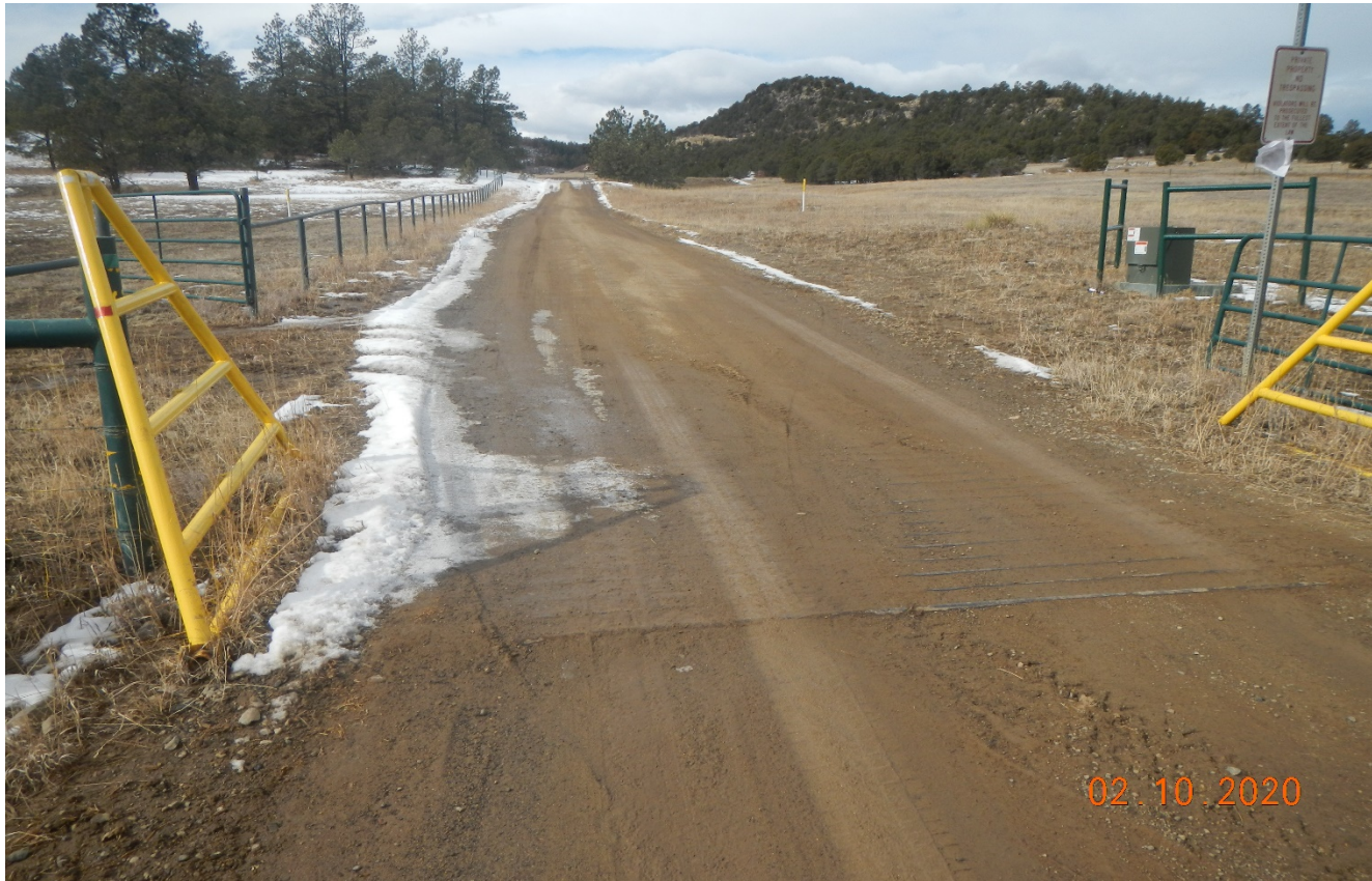
Photo 1. The cattle guard at the beginning of the access road is filled in with sediment.
