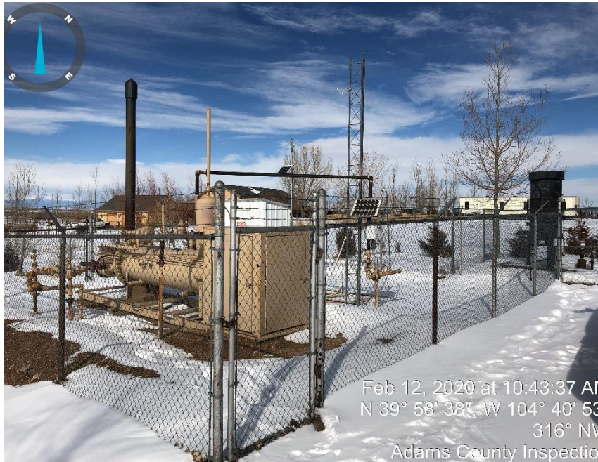
Photo #3 separator, meter run, RTU & combustor
