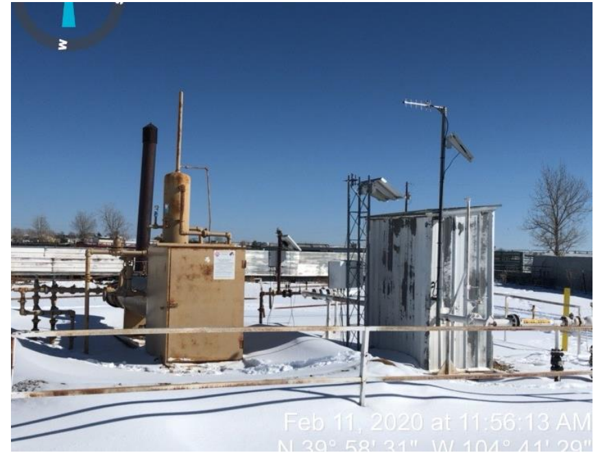
Photo #2 separator, RTU and meter run
